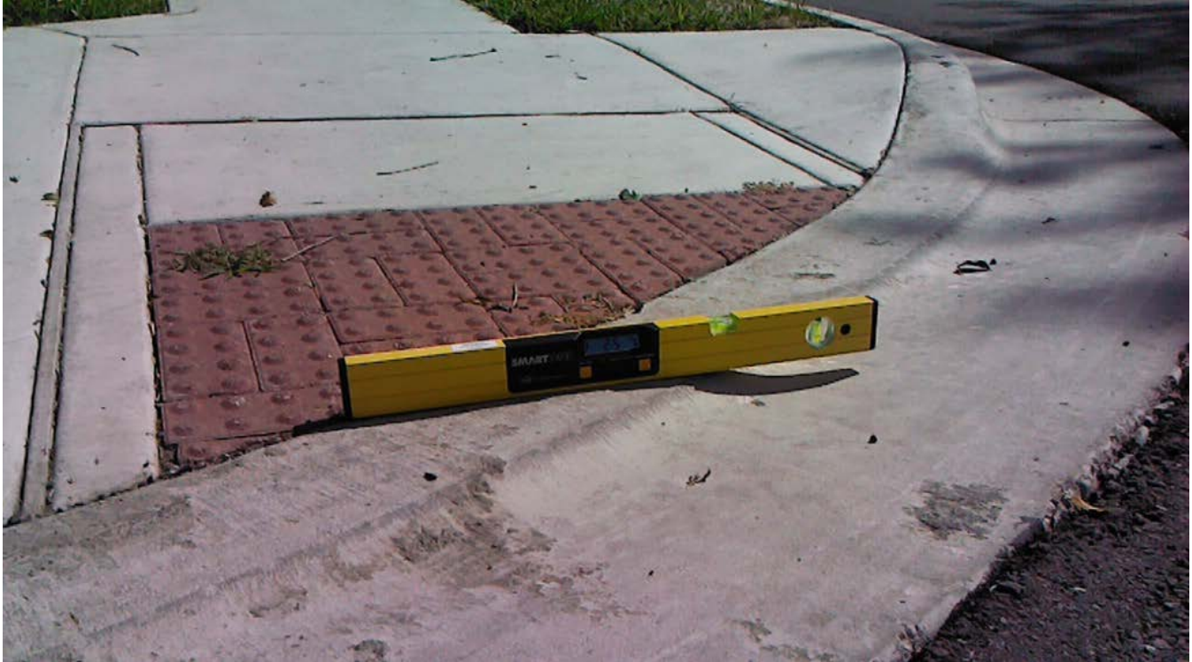
Figure 8. Curb Lip Fault (Formed/Constructed)
