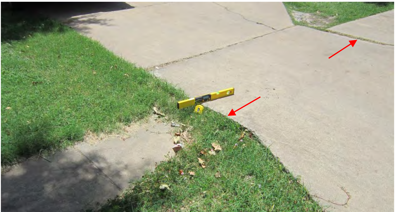
Figure 4. Sidewalk Faults at Driveway Interfaces
