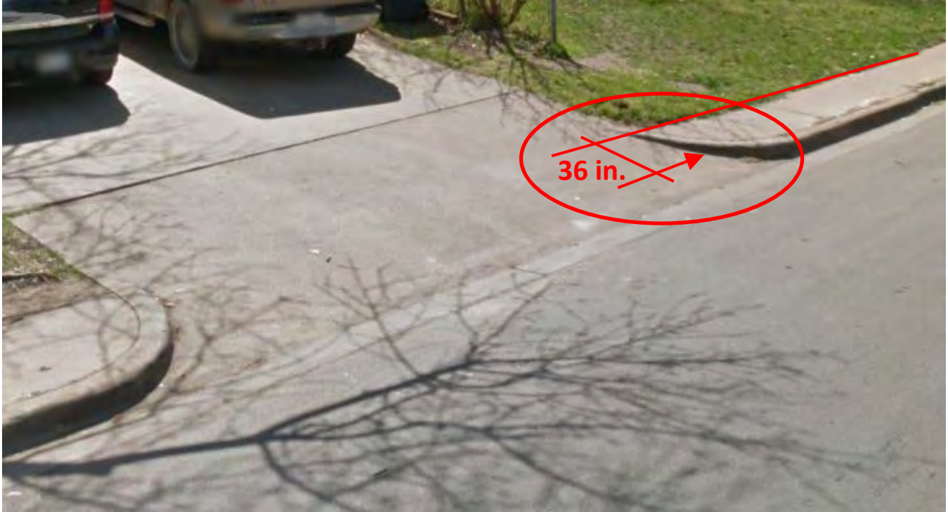
Figure 5. Returned Curb Fault (curb/fault height measured 36 in. from back edge of sidewalk)
