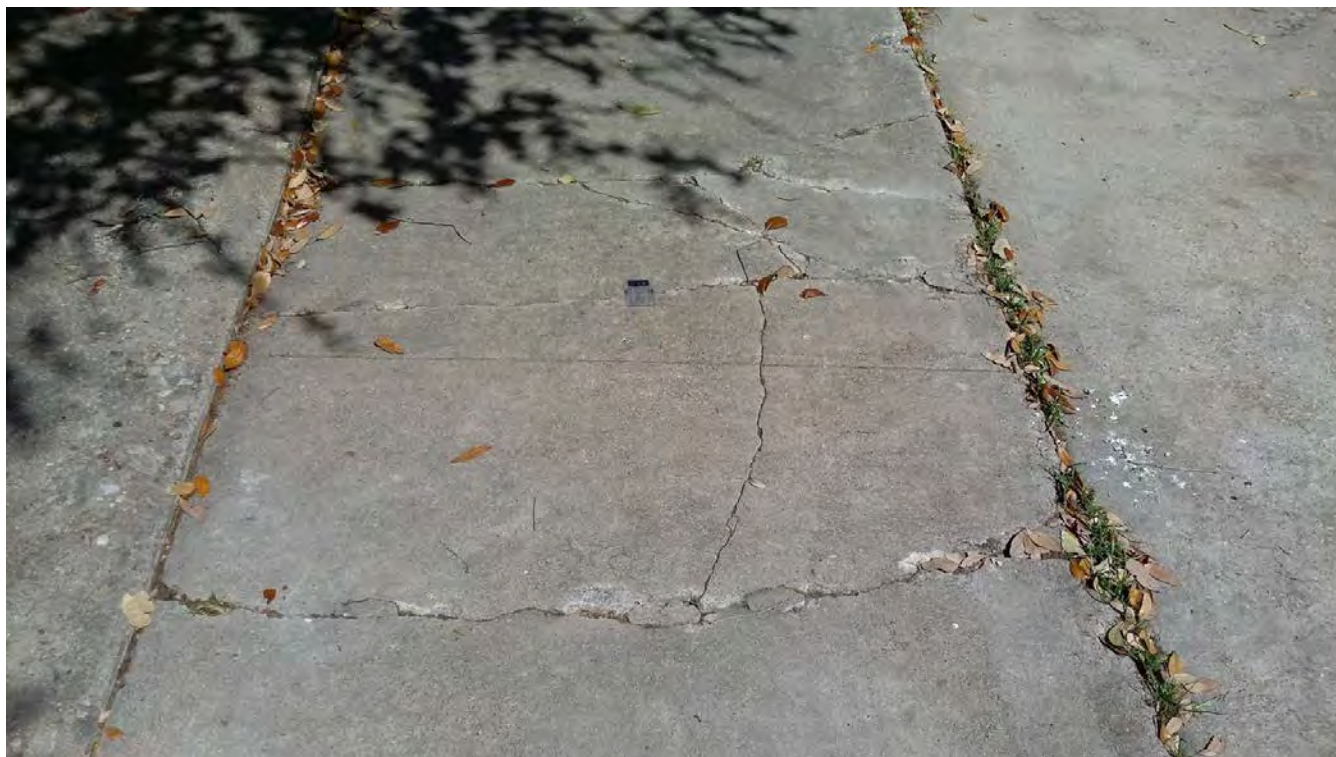
Figure 1. Cracking Ex. 1: Severe
