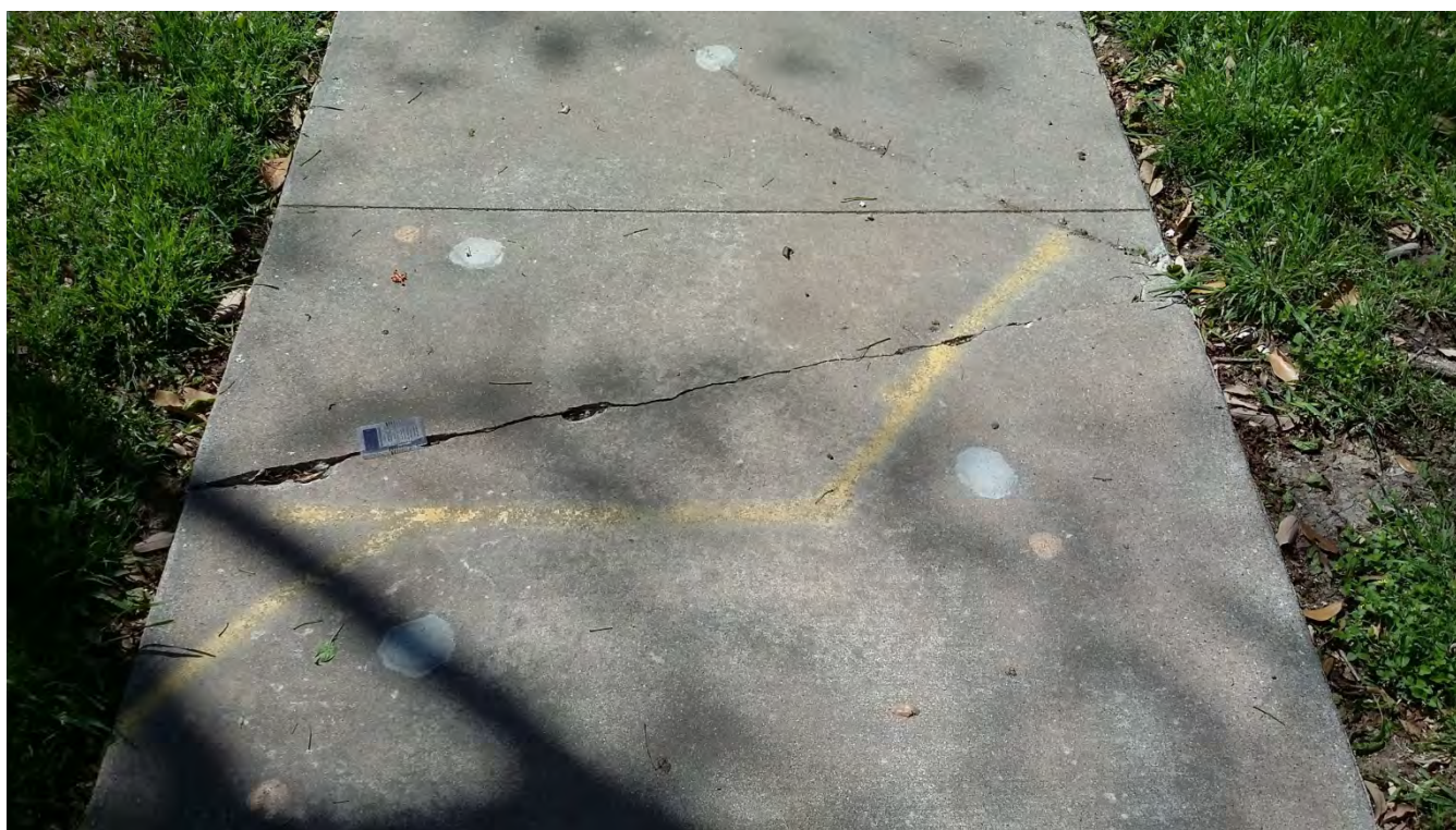
Figure 2. Cracking Ex. 2: Moderate
