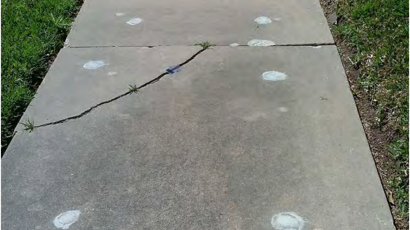
Figure 3. Cracking Ex. 3: Moderate
