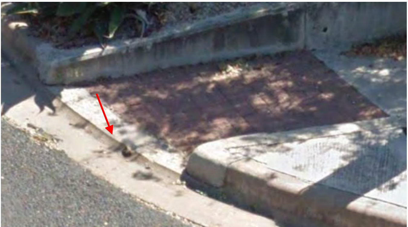
Figure 7. Curb Lip Fault (Sawed)
