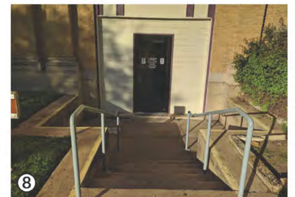
8 inaccessible entrance at southeast corner of main building: providing ADA access to this entrance from the nearby bus stop would be a positive side effect of lowering the lawn at the southern courtyard
