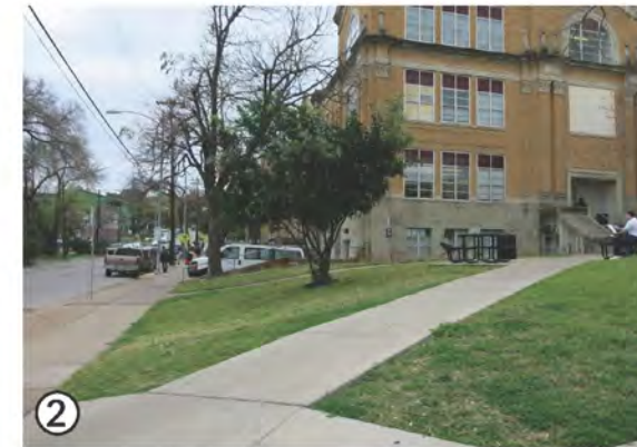
2 south-west corner of building: note the ADA non-compliant grading and existing West Street streetscape conditions, including dense overhead utilities & poles amongst trees, loading ramps, & generally cluttered condition
