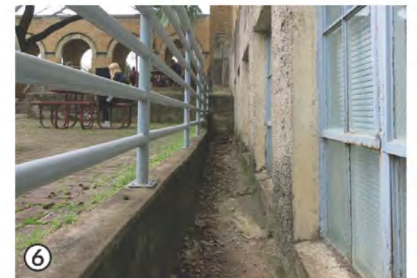
6 sunken light-wells at building face: storm water and debris collection an issue here, ensuring adequate drainage below the windows to help keep water away from the building will be crucial
