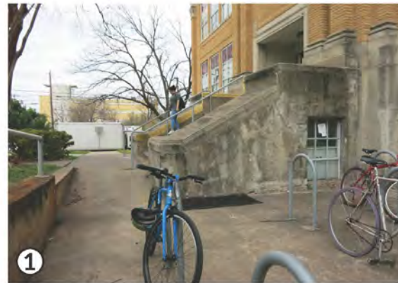
1 south-west entry stairs: note ramped condition at bottom of stairs and the relationship of the window to the elevation of the adjacent finished grade, floor (0) is 5' below bottom of window sill pictured here
