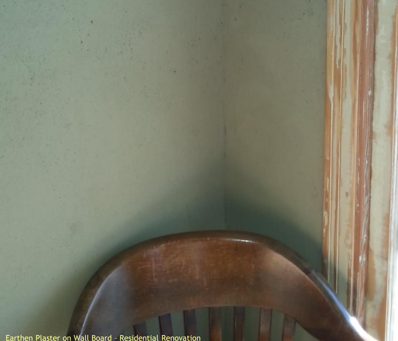
Earthen Plaster on Wall Board - Residential Renovation
