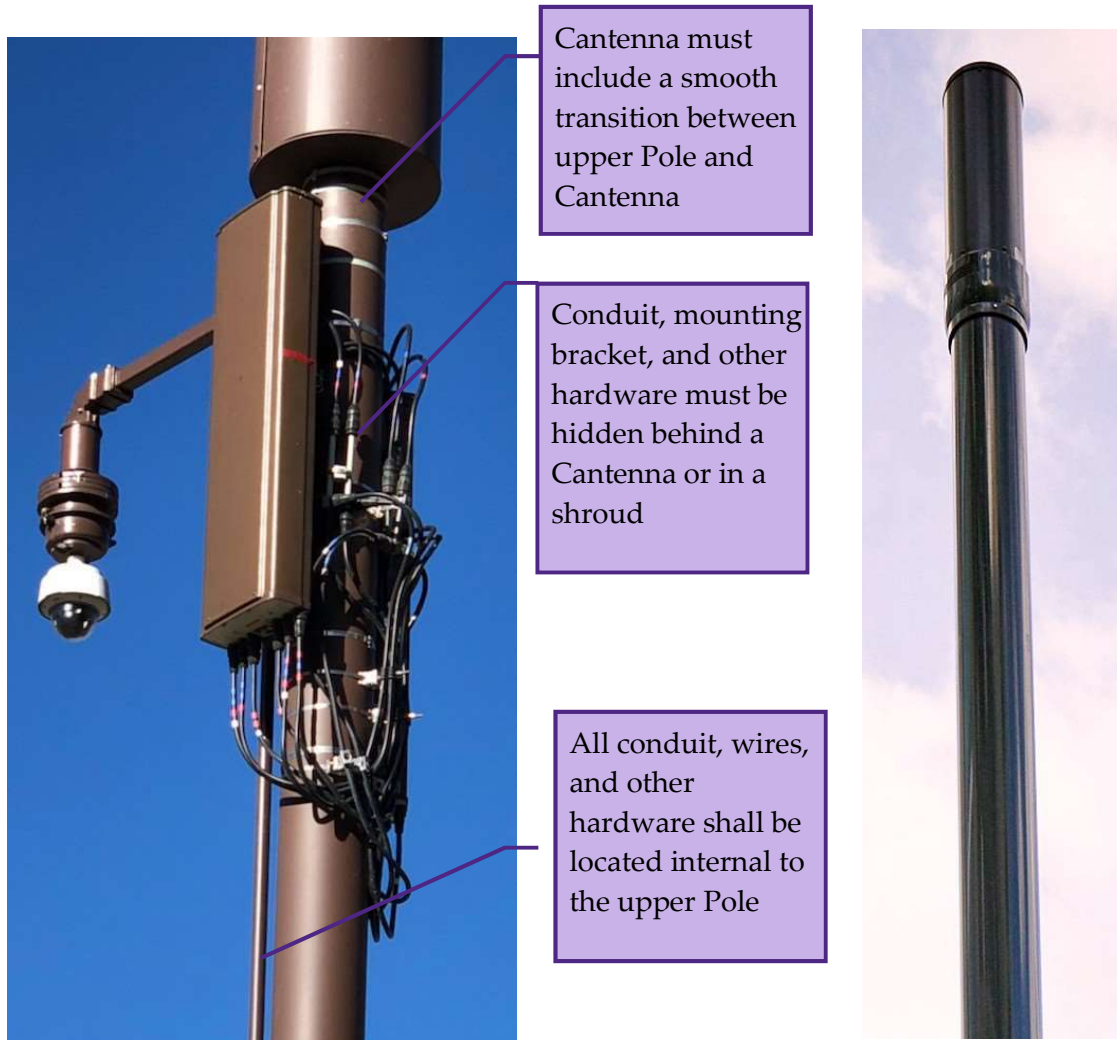
Figure 6-1: Unacceptable SC-3 Installation (L) and acceptable SC-3 installation (R)
