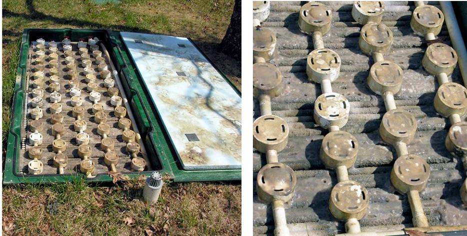
**Photograph 5: AdvanTex<sup>®</sup> System Receiving Residential Effluent with Water Softener Backwash Brine**
