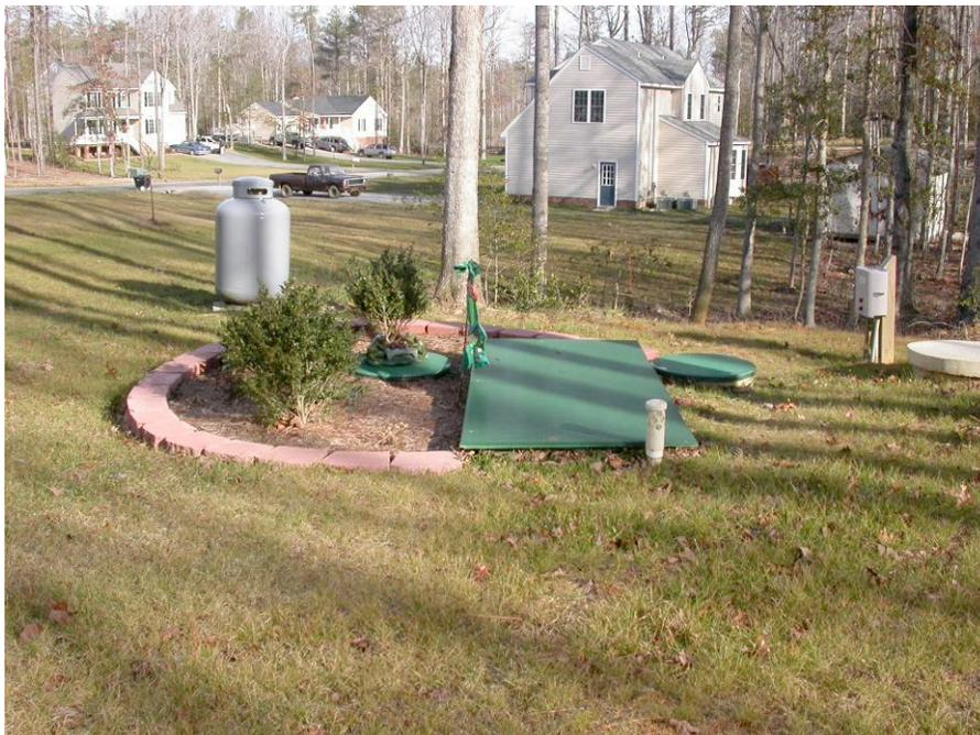
**Photograph 1: Typical AdvanTex® Installation**
