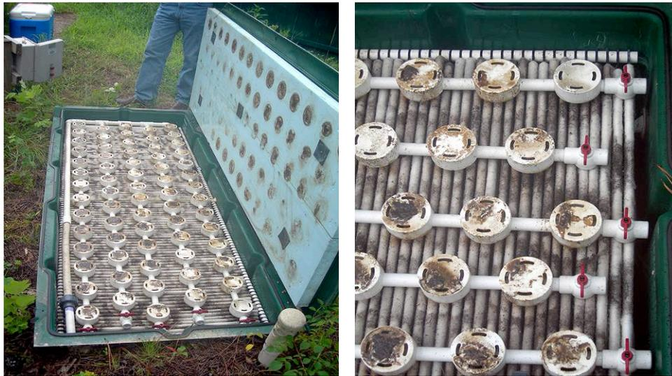
**Photograph 6: AdvanTex<sup>®</sup> System Receiving Residential Effluent with No Water Softener Backwash**
