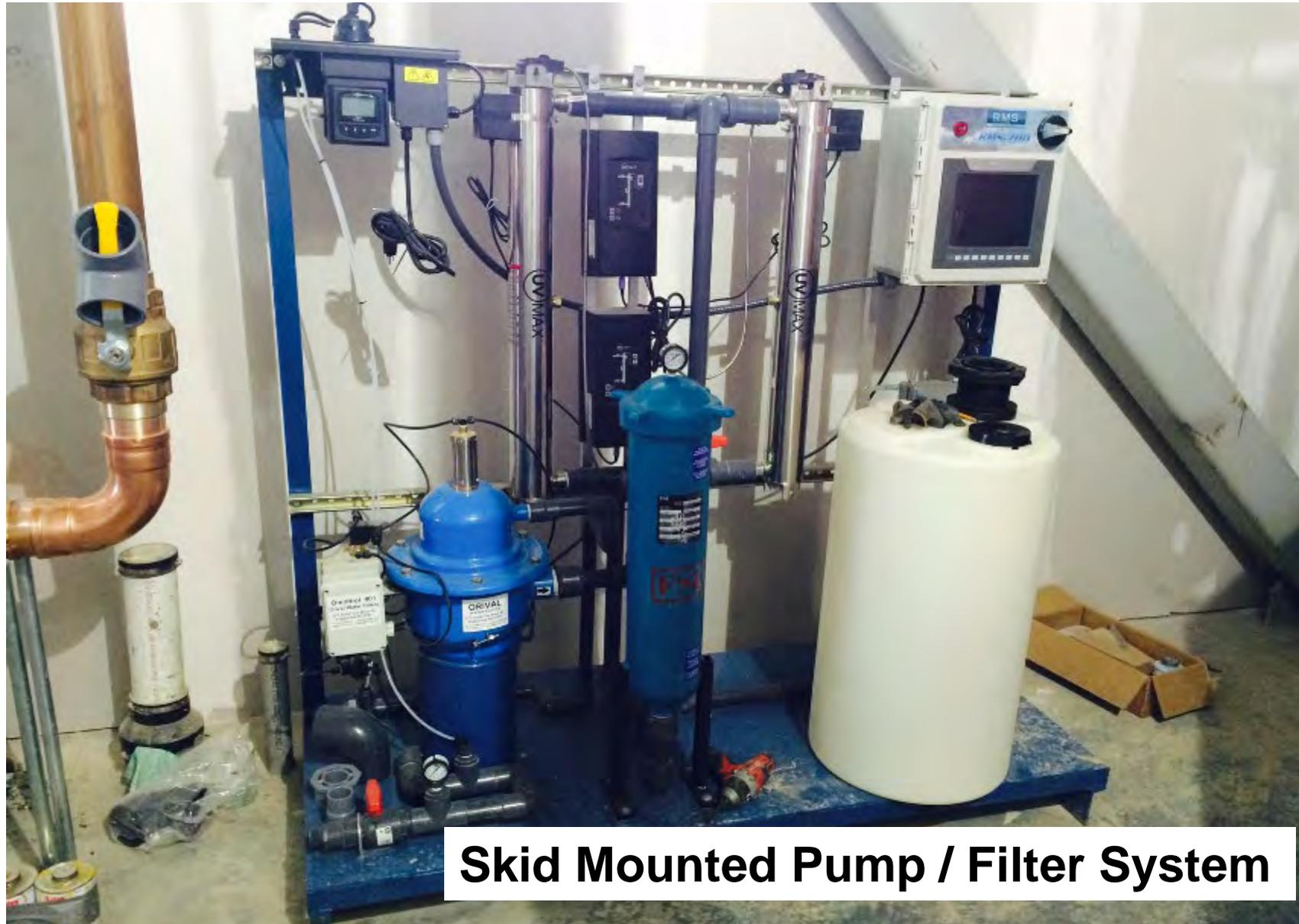
**Skid Mounted Pump / Filter System**
