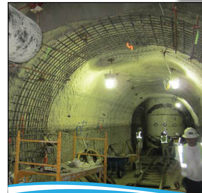
Left: Completed tie-in into Lake Travis raw water intake.
