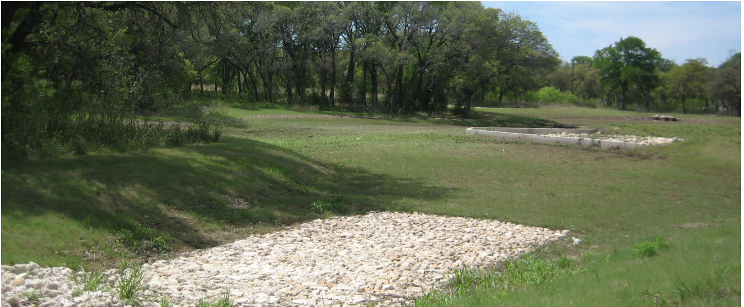
Lundelius McDaniels sedimentation basin and biofiltration pond.
