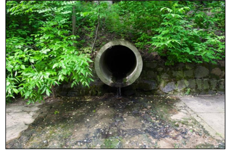
3. Rain water is released into the creek at the outfall. Sometimes it goes to a water quality or detention pond first.
