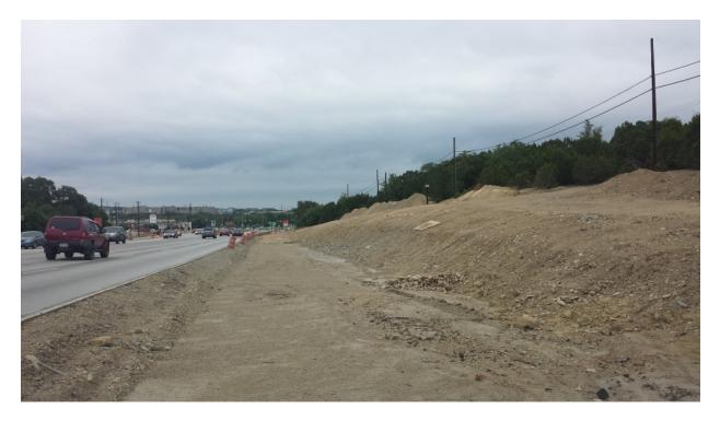
Figure 22 - US 290 Eastbound near intersection with SH 71 5-13-14. No temporary stabilization, no controls.
