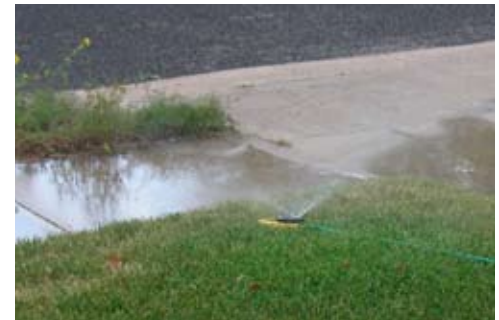
Manual sprinklers should also be placed correctly to avoid overspray
