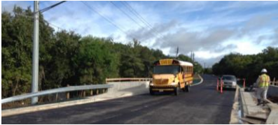
Low Water Crossing Upgrade
