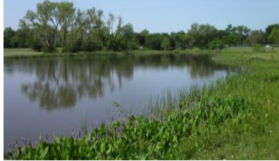
Regional Detention Pond
