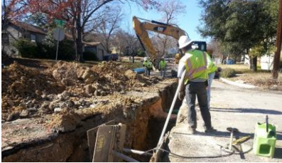
Storm Drain Improvements
