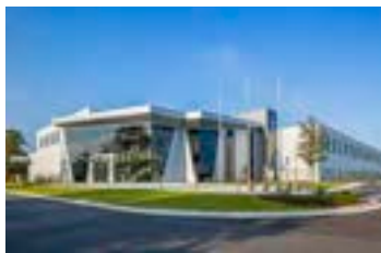
ROLLS ROYCE FACILITY SAVANNAH, GEORGIA $16,000,000
