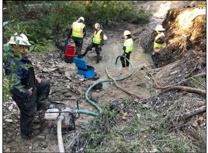
Figure 7. Multiple pumps are recommended for large pools to expedite the drawdown time
