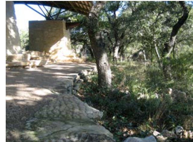
The South bathhouse should revel in its natural setting. Central Texas limestone should be strongly encouraged as the dominant building material.
