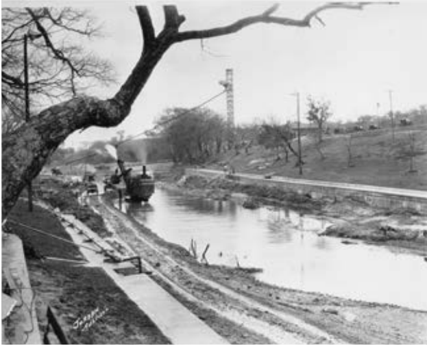
Barton Springs Pool under construction in the 1920s. C01818, Austin History Center, Austin Public Library.
