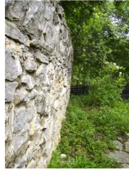
Photo 4: Retaining wall below medium tree well and west of spring
