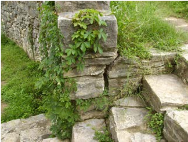
Photo 8: Inside wall of a typical stair.
