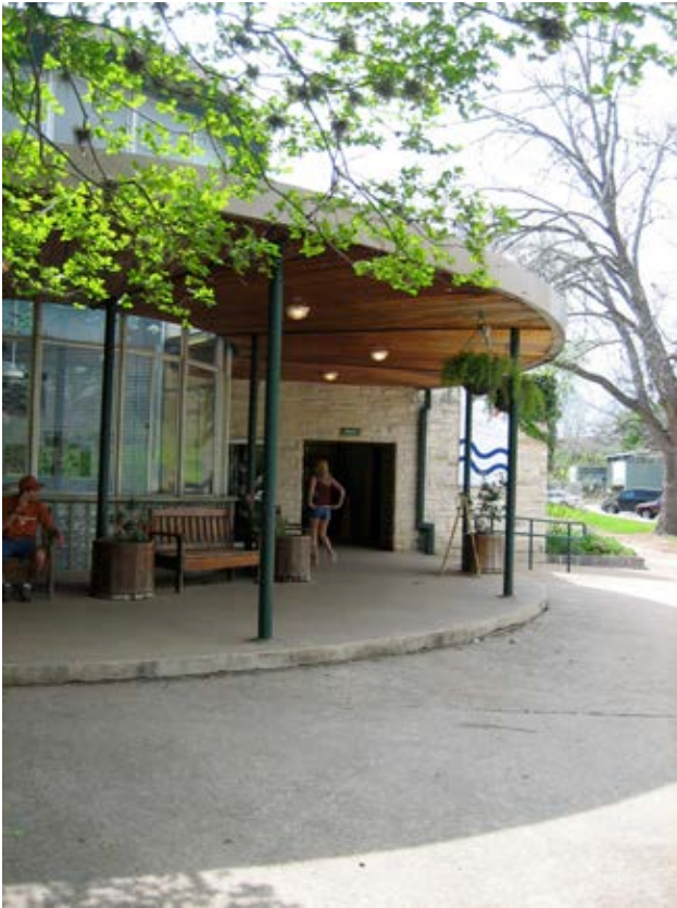
Existing 1947 Bathhouse. Originally, tickets were sold through ticket windows in the glass rotunda.
