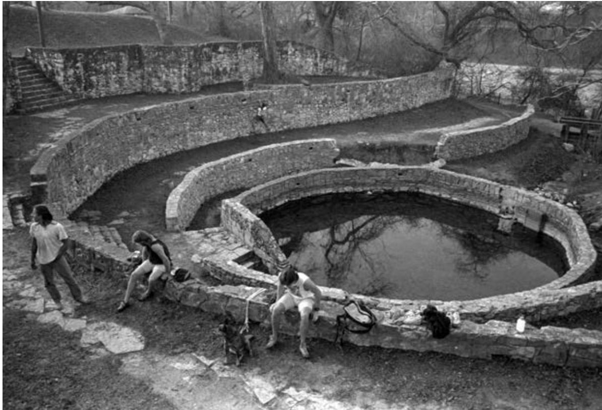
A dozen years later, Sunken Garden on February 19, 1993. The landscape is still nicely groomed and the flagstone paving stones are not yet obscured by overgrowth. According to photographer Alan Pogue, the wall section collapsed in the flooding of 1991. Note that the wall section to its right appears to be leaning as does the wall above it. Photo: Alan Pogue
