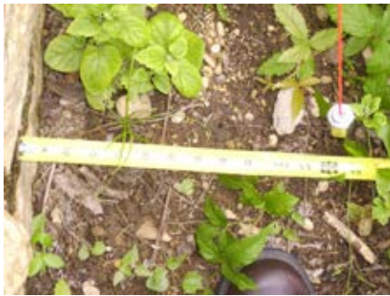
Photo 5: Retaining wall below medium tree well and west of spring
