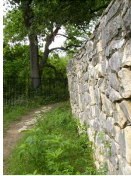
Photo 3: Retaining wall west and below large tree well
