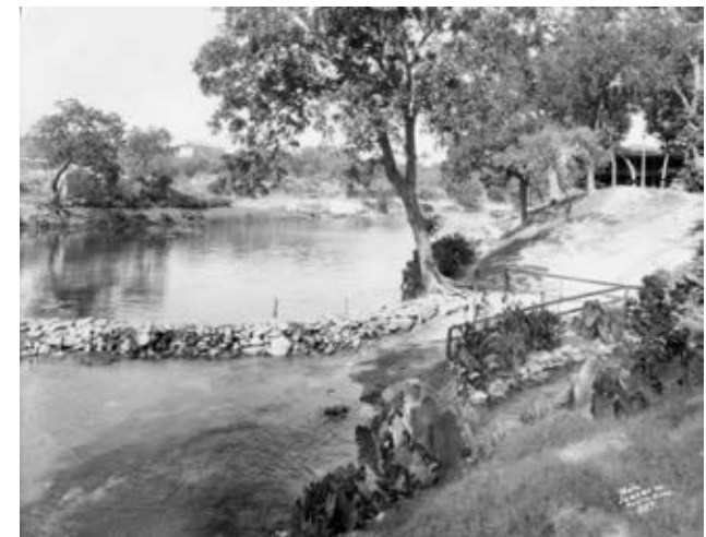
Barton Springs Pool, circa 1925. Prior to the construction of the permanent dam, temporary rock dams were built each spring to make the pool. C01803, Austin History Center, Austin Public Library.
