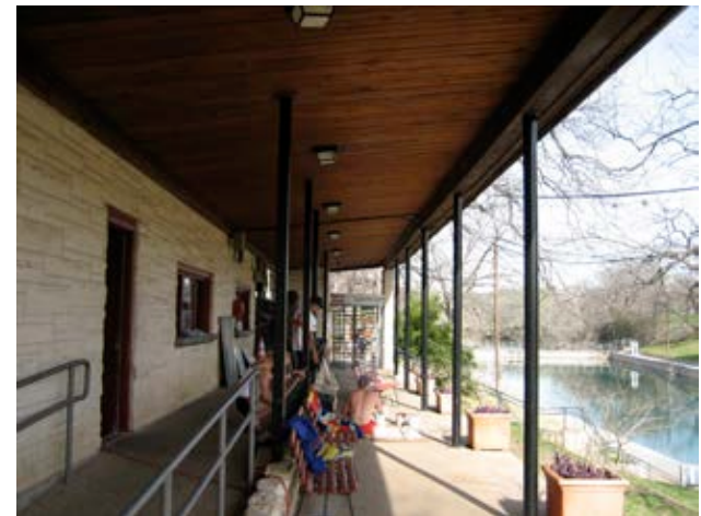
The relocation of the Lifeguard's Lounge/Manager's Office in the 1960s required this elevated passage to account for a level change, changing what was designed to be a shaded social space into more of a passageway.
