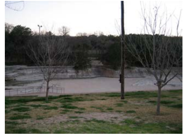
Newly planted trees benefit from separate irrigation from that provided by lawn sprinklers. New trees require irrigation for at least two years to become established.
