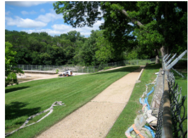
A sliver of grass atop a low retaining wall that is awkward to mow. It is also used for very visible pool equipment storage.
