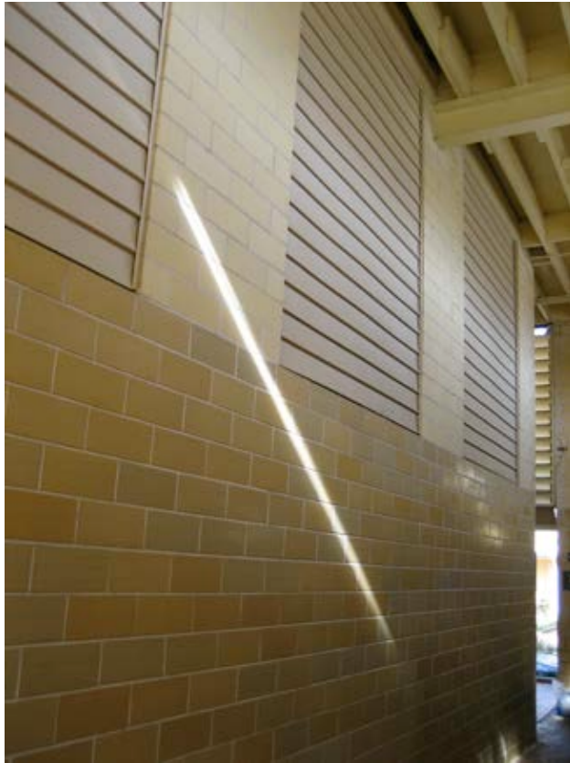
What were originally designed as generous openings into the basket rooms are covered with vinyl siding. A rehabilitated Bathhouse should replace the siding with glass to create a light-filled, double-height space.
