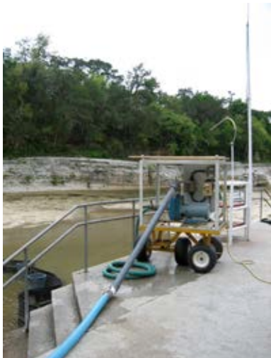
Trash pump used for silt disposal.
