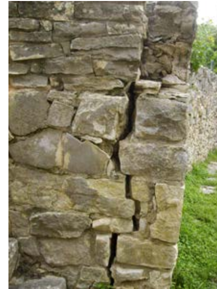
Photo 9: Inside wall of a typical stair.
