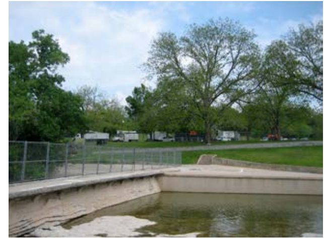
The fencing at the dams must be easy to remove, durable, and inexpensive to replace when it gets damaged.
