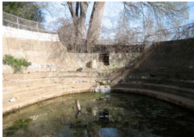
View towards Pool. Stonework should be removed to reopen slot in amphitheater, allowing flow into recreated spring run.
