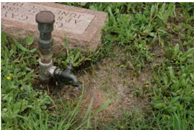
Figure 387. Ponding water in Section A (McDoux Preservation)
