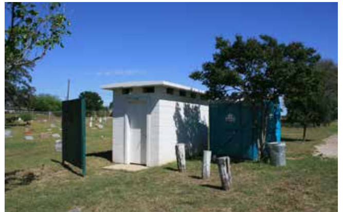
Figure 404. The small restroom facility and adjacent portable toilet (John Milner Associates)
