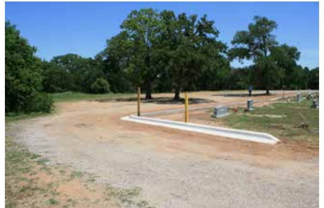
Figure 354. A concrete curb lines a portion of Avenue K to prevent damage to headstones from vehicles. This street has since been repaved. (John Milner Associates)
