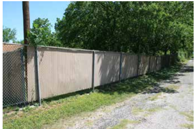
Figure 407. Screening elements installed on the chain link fence by adjacent property owners (John Milner Associates)
