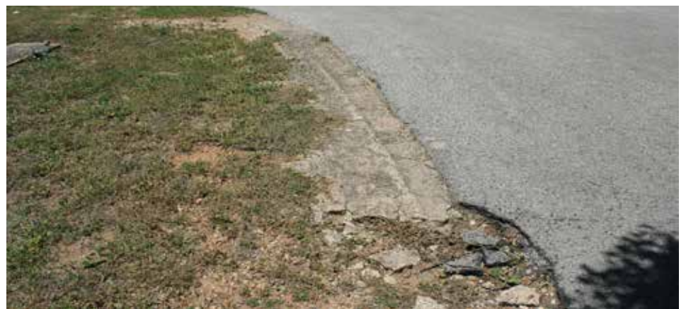
Figure 355. Edge degradation of the cemetery drive due to vehicle parking (John Milner Associates)
