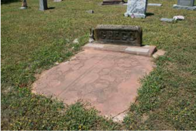
Figure 394. Formal plot coverings include this example of a stamped concrete slab. (John Milner Associates)
