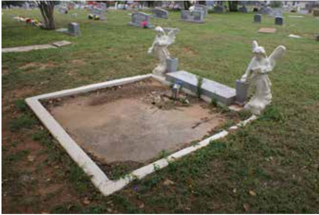
Figure 400. Concrete curbing enclosing a plot (McDoux Preservation)
