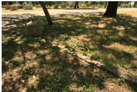
Figure 410. A concrete curb in Section C terminates in a concrete litter receptacle. (John Milner Associates)
