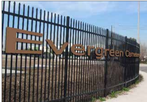
Figure 418. Example of a sign on a curved black metal picket fence (Google, annotated by John Milner Associates)
