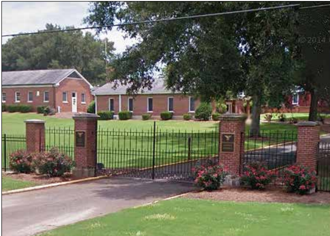
Figure 424. At Andersonville National Cemetery, brick columns support a traditional black picket fence. (Google)
