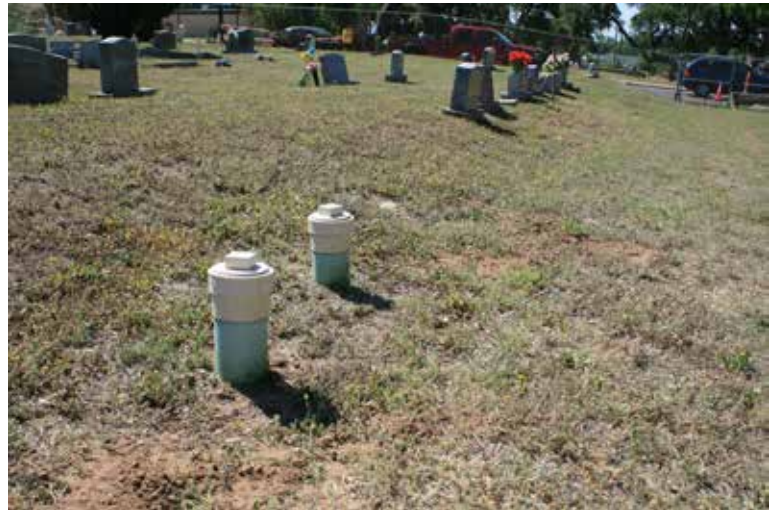
Figure 416. PVC sewer standpipes near the location of the former caretaker's house (John Milner Associates)
