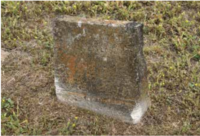
Figure 383. The base of this marker is heavily damaged by trimmers (McDoux Preservation)
