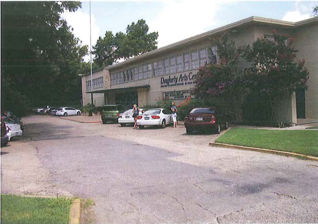
1. South façade of the Dougherty Arts Center, facing Barton Springs Road. In general, this façade preserves the original appearance of the 1947 Naval and Marine Reserve Center.
