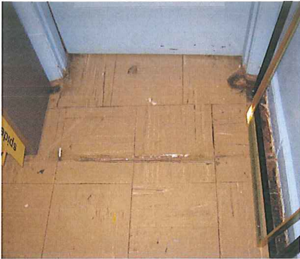
20. Slab and tile conditions in Area E (13N).
