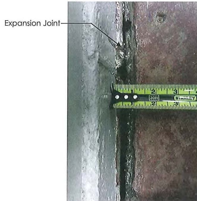
Photo 1: Expansion joint between perimeter grade beam and slab
