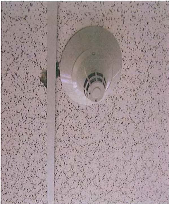
7. Evidence of raccoon infestation in Area A (202W).
