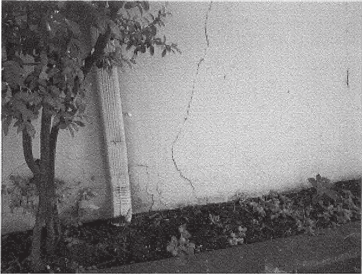
30. Typical exterior conditions of Area E.
