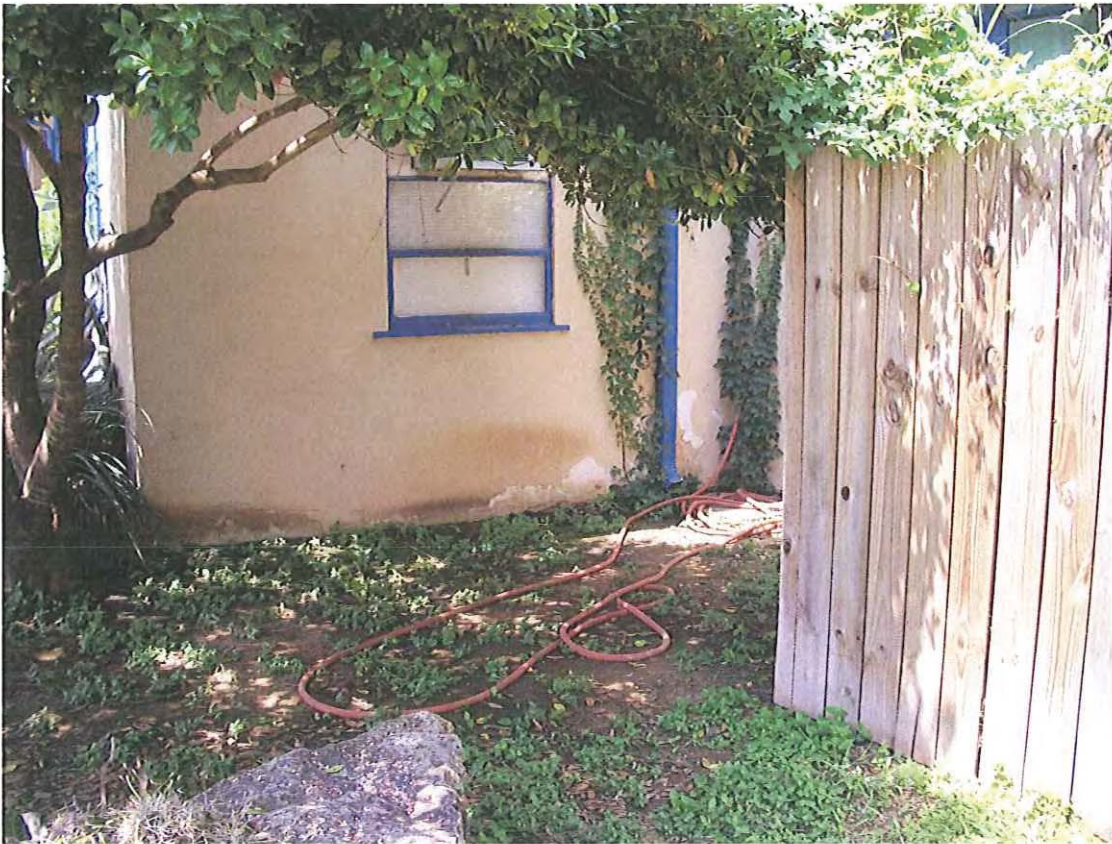
29. Typical exterior conditions of Area E.
