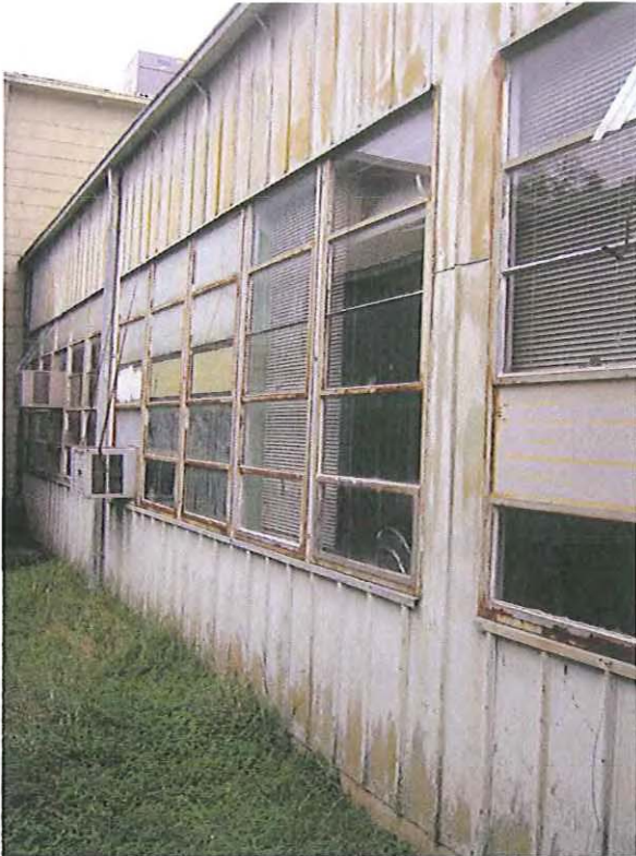
11 A/B. Exterior of East and West side of Area B. Presumed original metal windows and wall panels installed in 1947.
