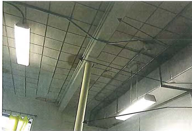
Photo 9: Water damage in ceiling
