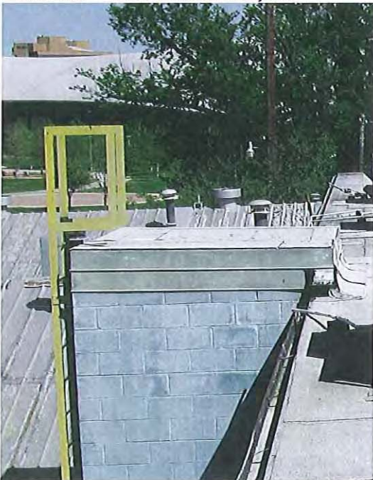
Photo A-5.1 Flashing weathered, but functional.
