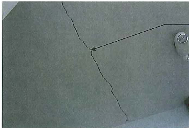
Photo 7: Cracks in gypsum board
