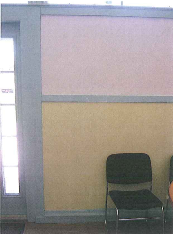
22. Interior conditions in Area E.
