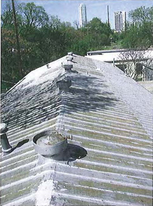
Photo B-1.1 Looking North.
