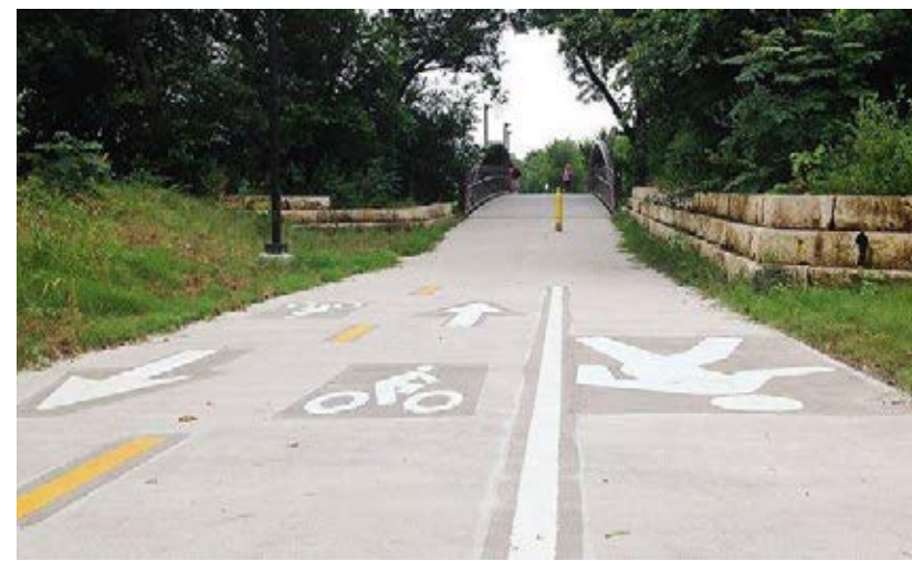
A View of newly-constructed bicycle & pedestrian bridge crossing of Boggy Creek, looking north
