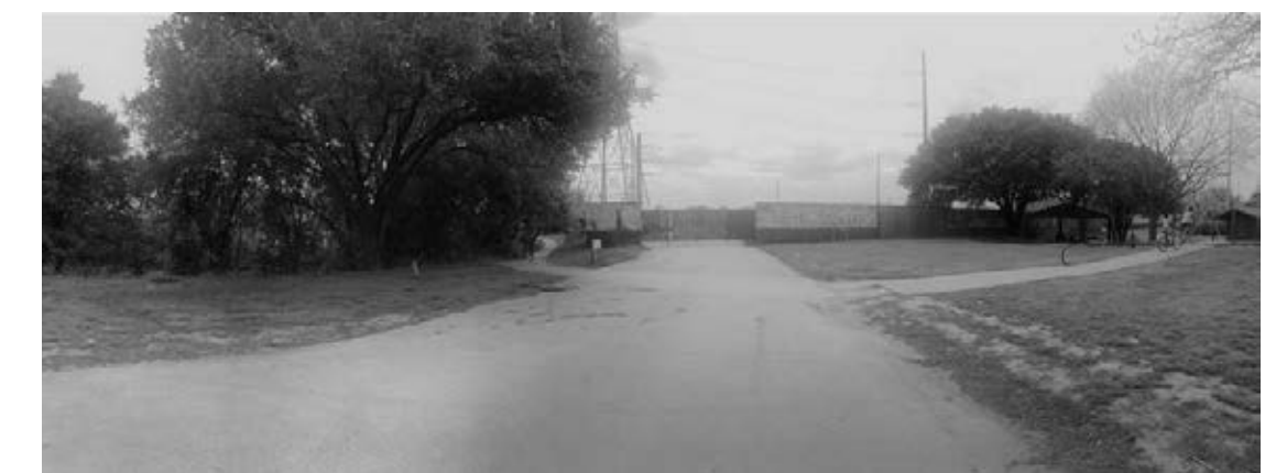
Existing view of the former Holly Street Power Plant walls, looking south toward Lady Bird Lake
