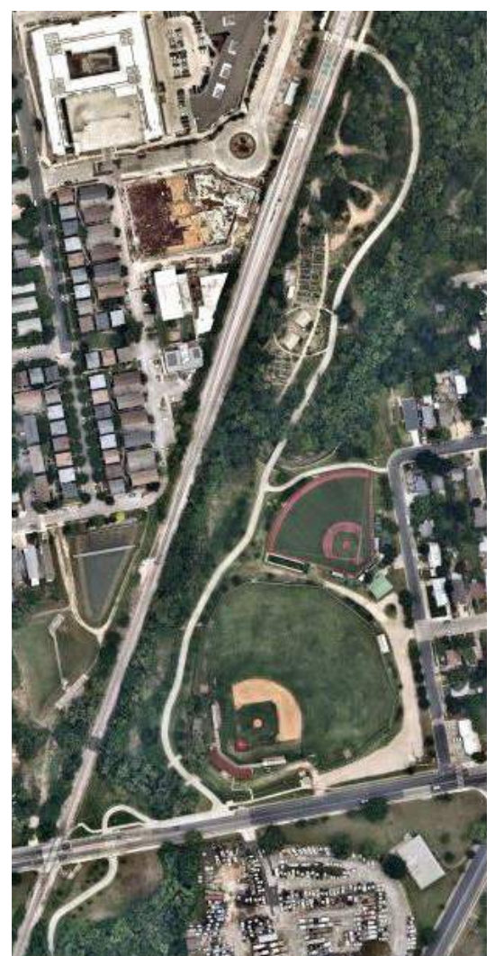
View of recently-completed shared use path and bridge improve connectivity along Downs-Mabson Fields and the Sustainable Food Center’s Community Gardens. (NearMap, 2020)
