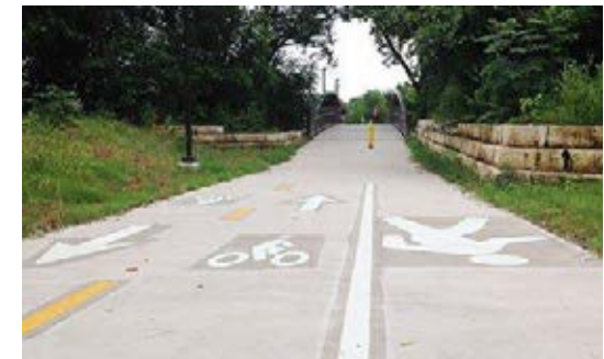
View of newly-constructed bicycle/pedestrian bridge crossing of Boggy Creek, looking north
