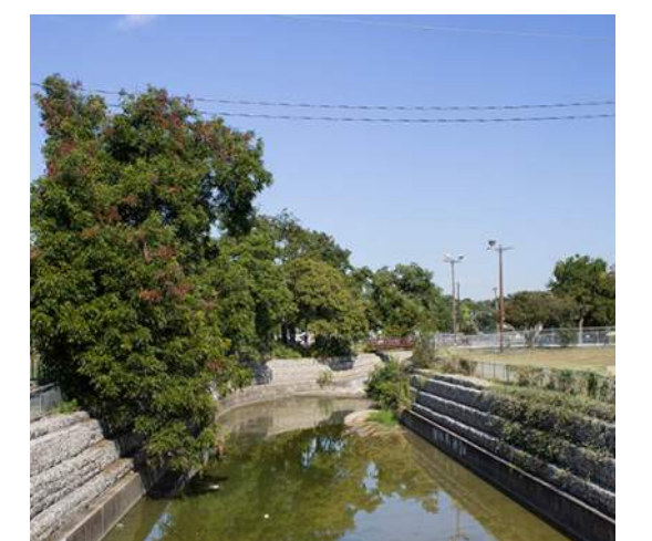
Boggy Creek channelization at Parque Zaragoza
