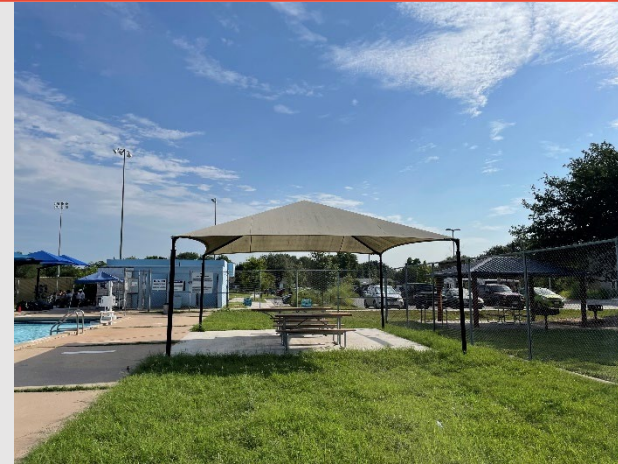
Fabric Shade Structure at East Lawn Cubierta de tela
