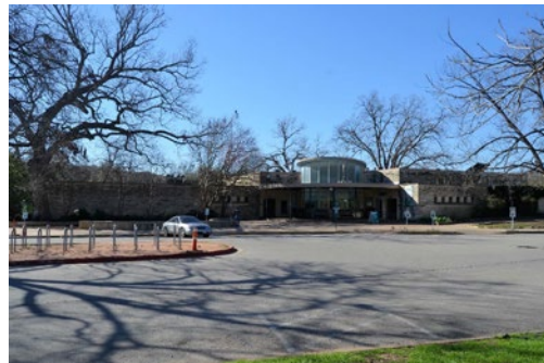
Zilker-Metro Barton Springs Bathhouse Rehabilitation
