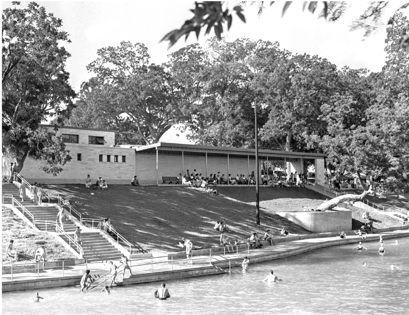
Barton Springs Bathhouse Rehabilitation
