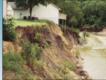
Little Walnut Creek at Bridgewater
