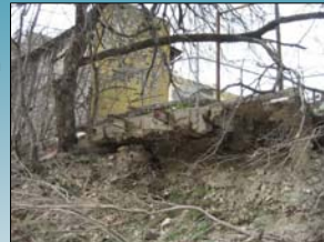
Right bank downstream of W 5th St.
