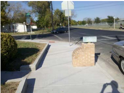
Johnston Terrace Safe Routes to School Sidewalk
