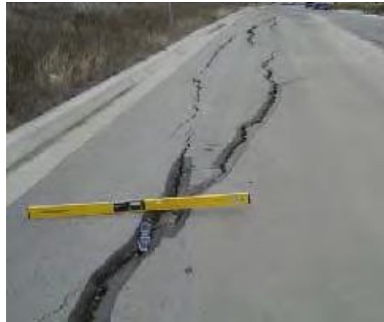
Left: Photo of pavement cracks in a new Austin subdivision in 2009. Right: Longitudinal cracking on Golden Falls Drive in Travis County in 2008. Photo credit: City of Austin.
