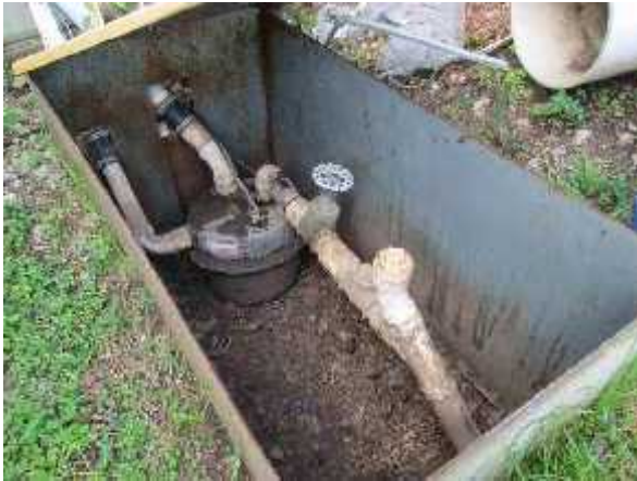
Photo 13 View of sump pump onsite
