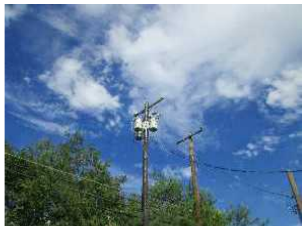
Photo 24 View of pole-mounted transformers onsite
