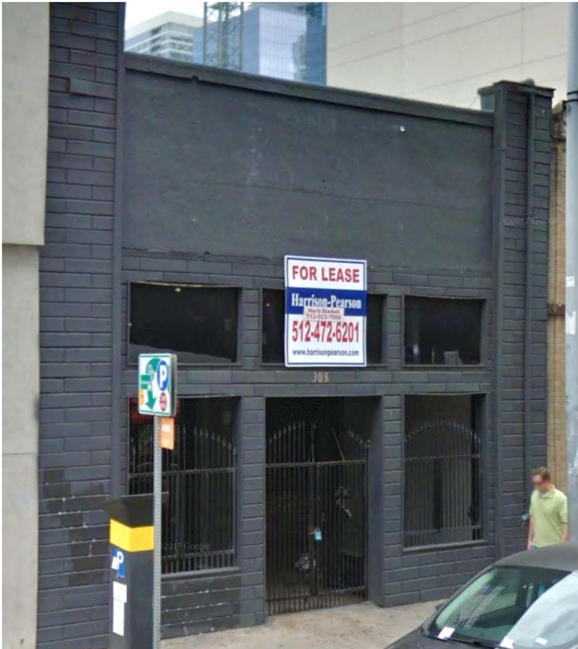
2017 photograph showing the painted stone treatment over the stucco shown in earlier photographs and the removal of the front part of the interior to create the enclosed courtyard
