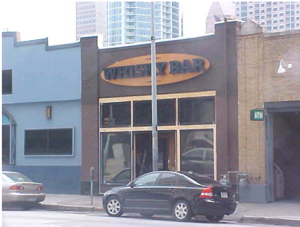
2008 photograph showing historic storefront
