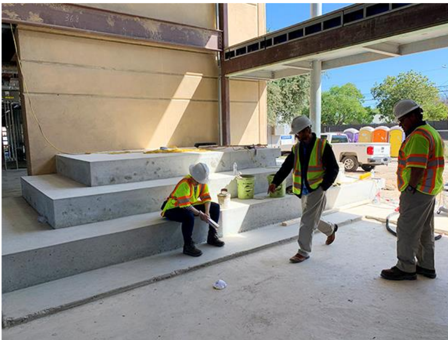
Lobby staircase/sitting steps concrete poured
