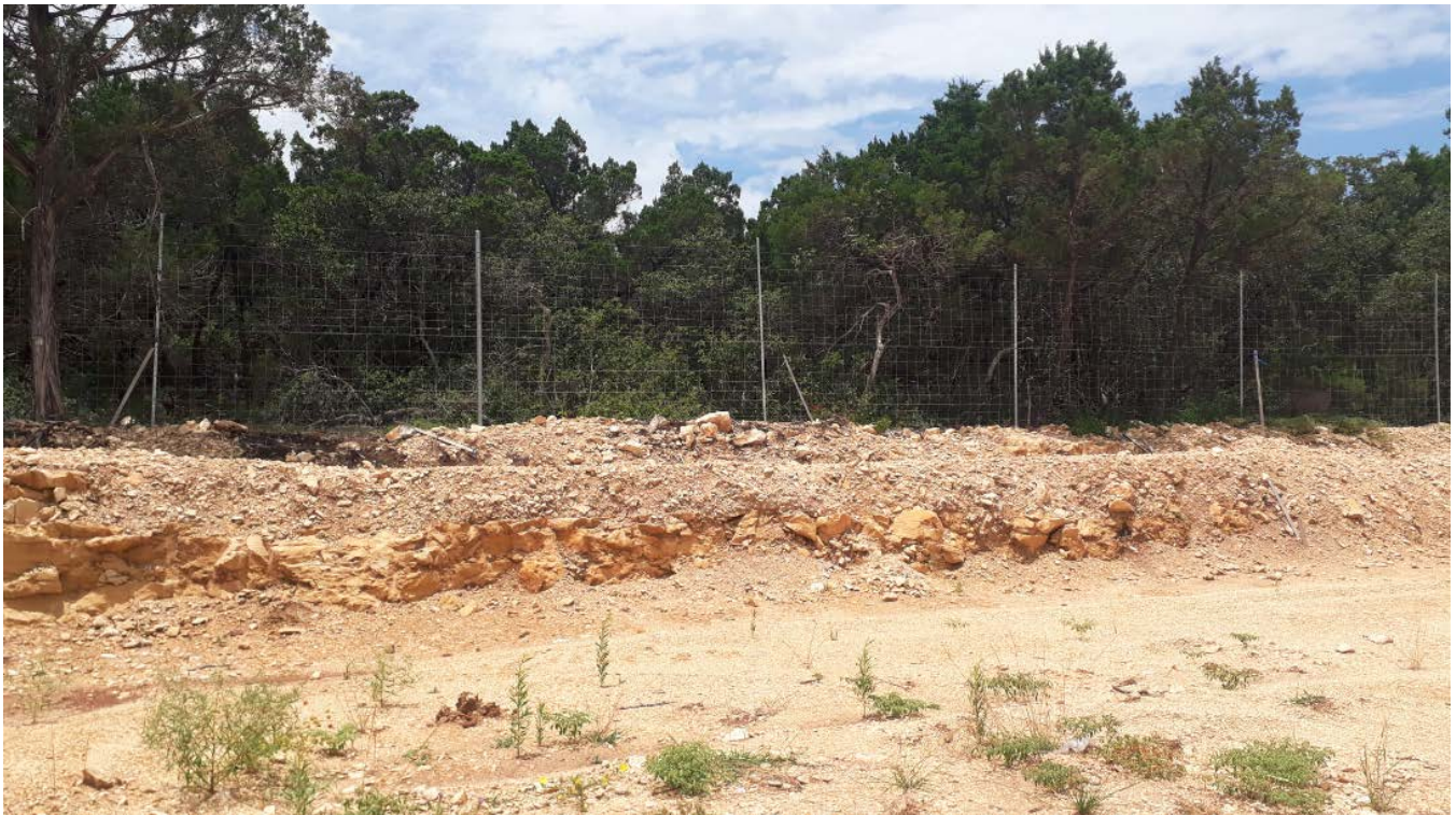
Figure 37. Down Cutting to Level Development Site Adjacent to Tooth Cave, June 2020
