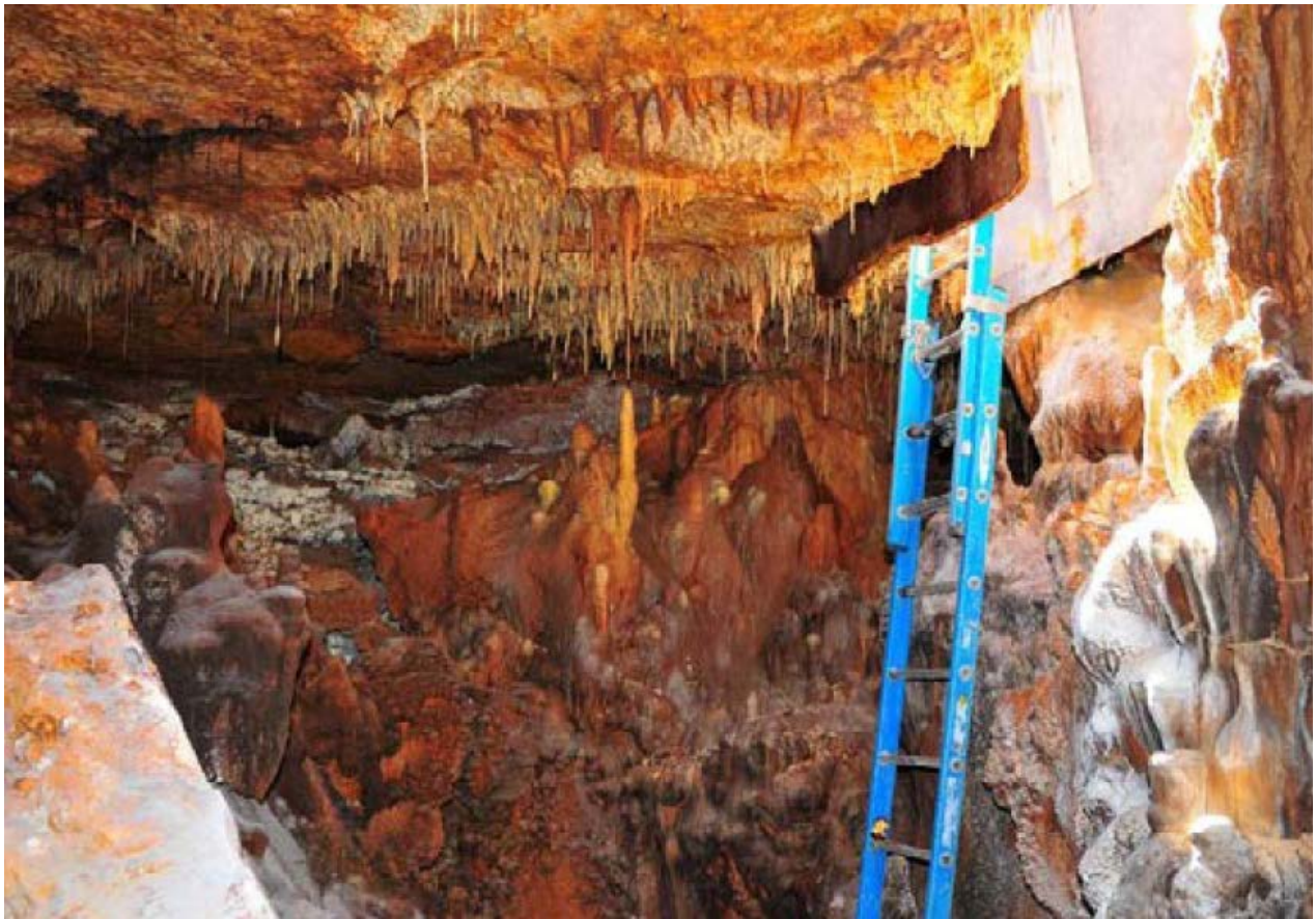
Figure 5. Cave “Void” Encountered by Trench in Austin Texas
