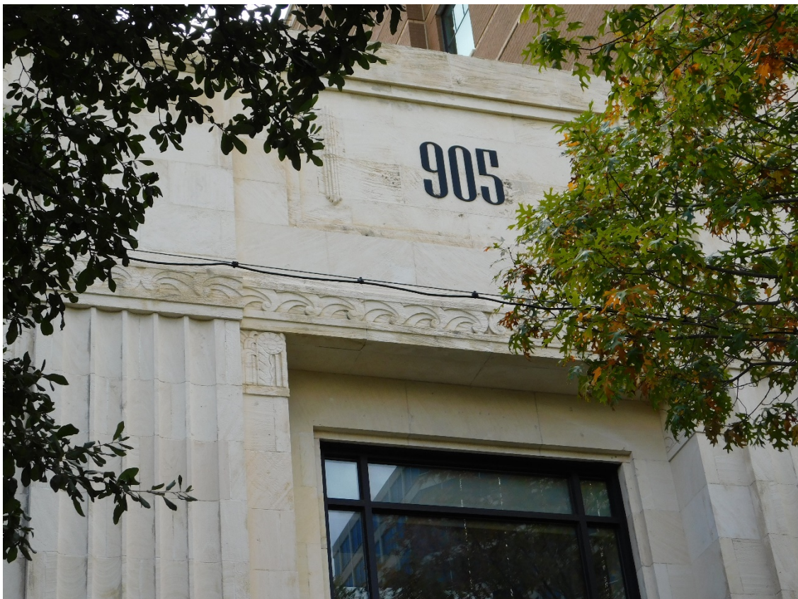
Detail of the fluted pilasters, the top of the central window, and the parapet, featuring a course of stylized wave motifs at its base.
