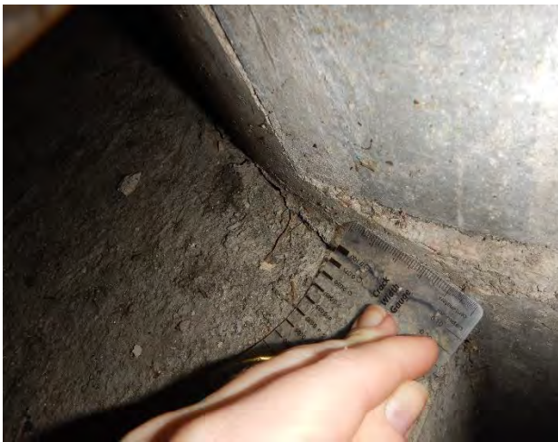
Figure 13. Column-to-ramp/slab perimeter crack.
