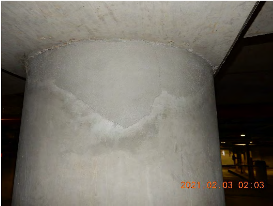
Figure 15. Previous column repair at intersection of slab.
