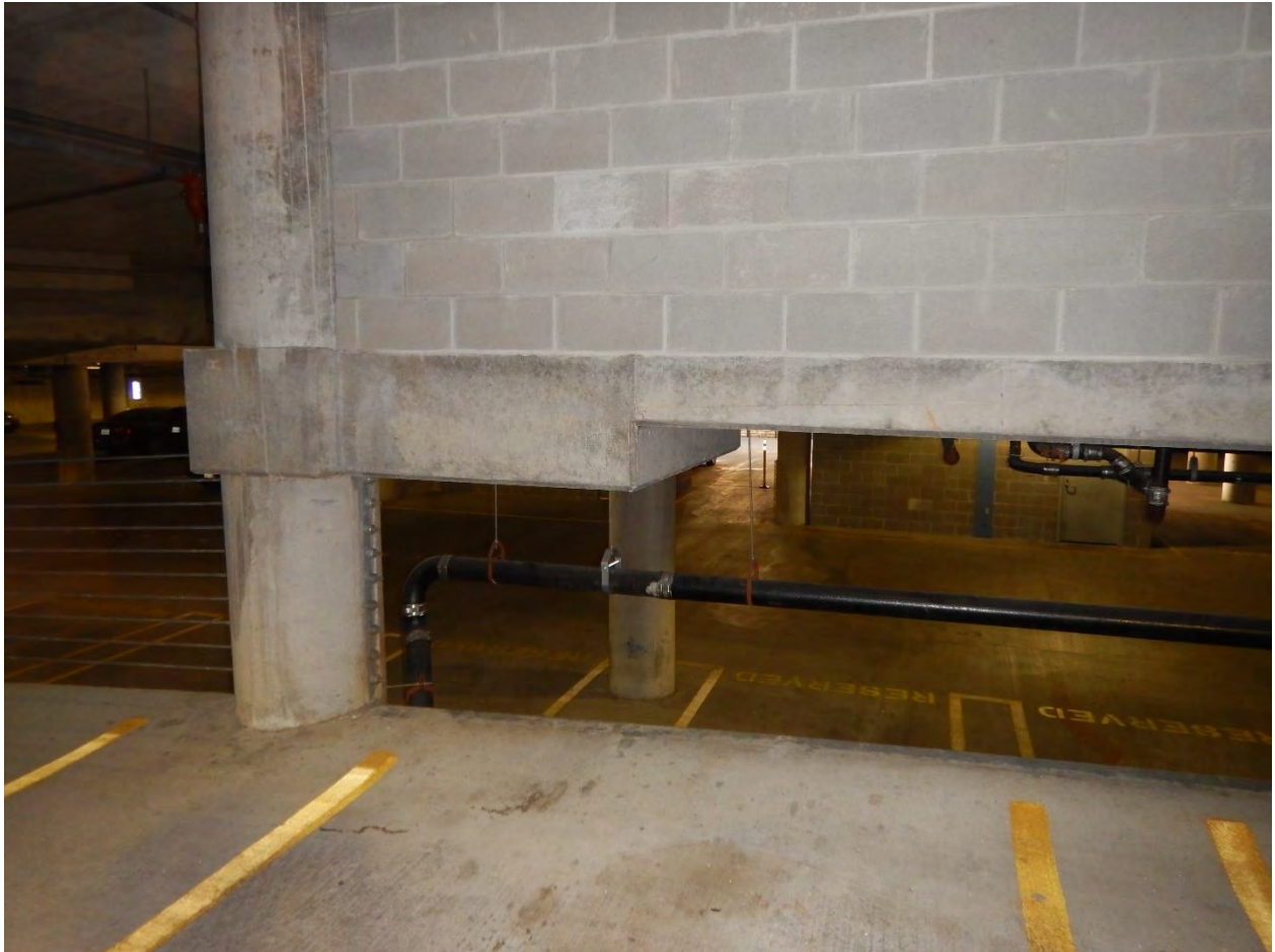
Figure 31. Ramp section without barrier cables.
