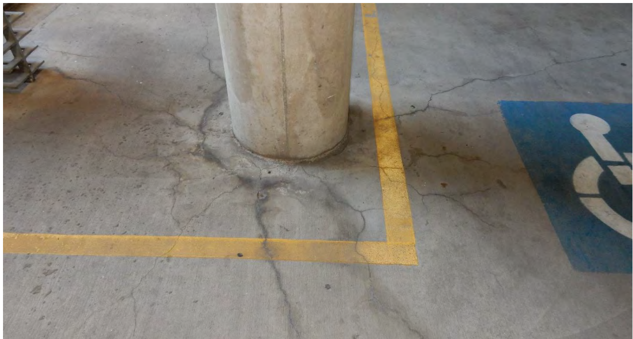
Figure 20. Observed radial cracking from columns.
