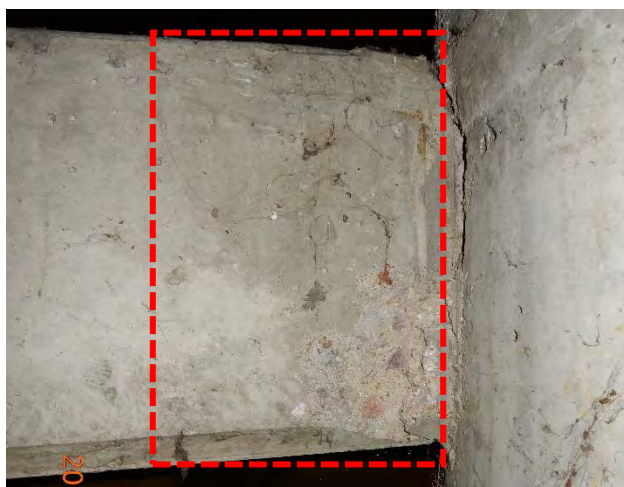
Figure 14. Column-to-ramp/slab interface vertical crack.
