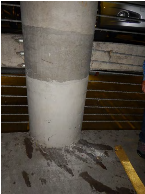
Figure 16. Previous column repair at intersection of ramp slab.
