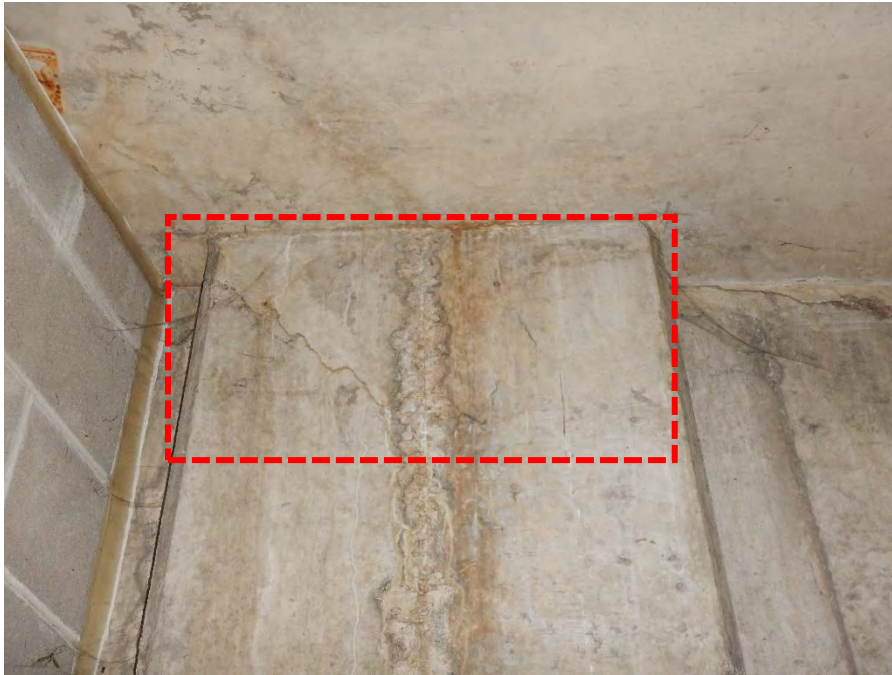
Figure 25. Delamination observed near the soffit of P1 adjacent to the ventilation chase (highlighted in red).
