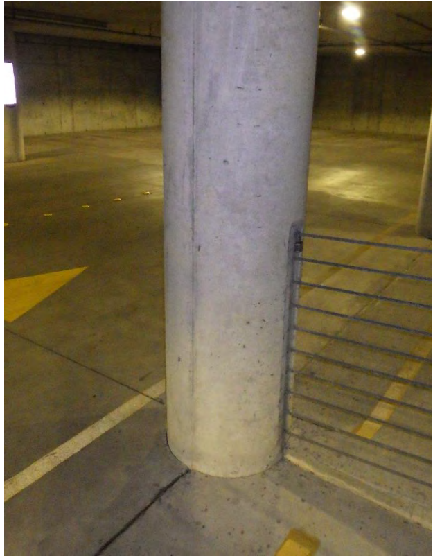
Figure 9. Column along Gridline 3.5 and 9.5 where floor slab and ramp slab intersect with column at the same elevation.
