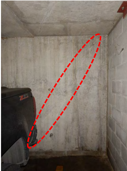
Figure 21. Typical diagonal crack observed in perimeter walls noted in red.
