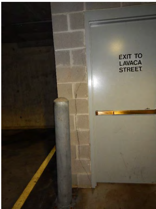
Figure 26. CMU cracking adjacent to wall opening.
