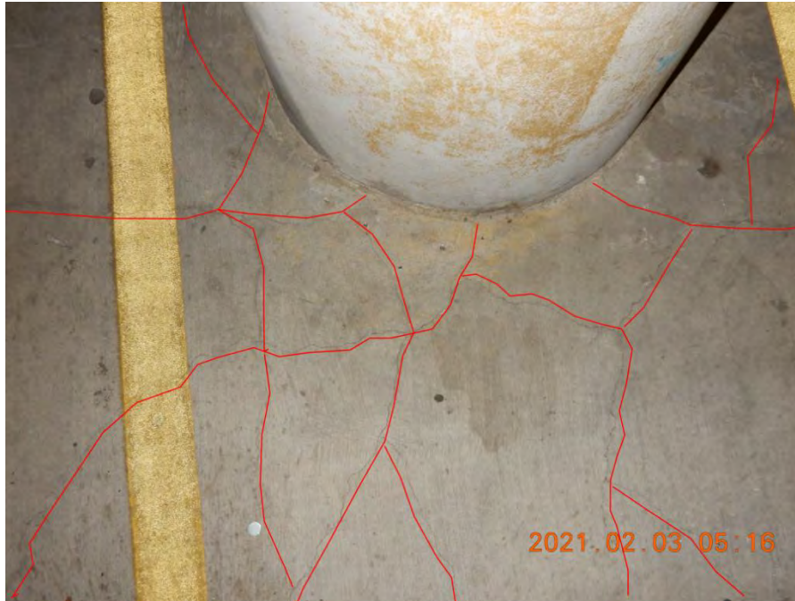
Figure 19. Slab radial cracking around column.
