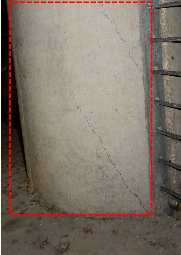
Figure 11. Column delamination (red) and cracks above the intersection slab.
