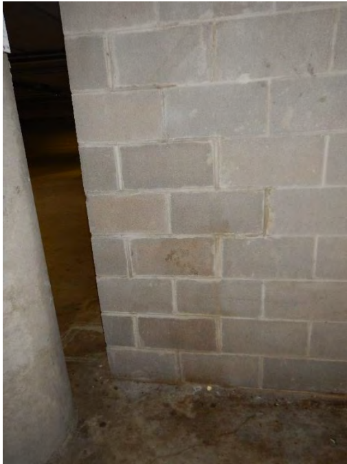
Figure 23. Evidence of previous CMU wall repair at wall intersection.
