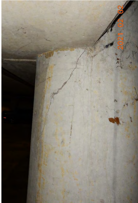
Figure 12. Column delamination and cracks below the intersecting slab.
