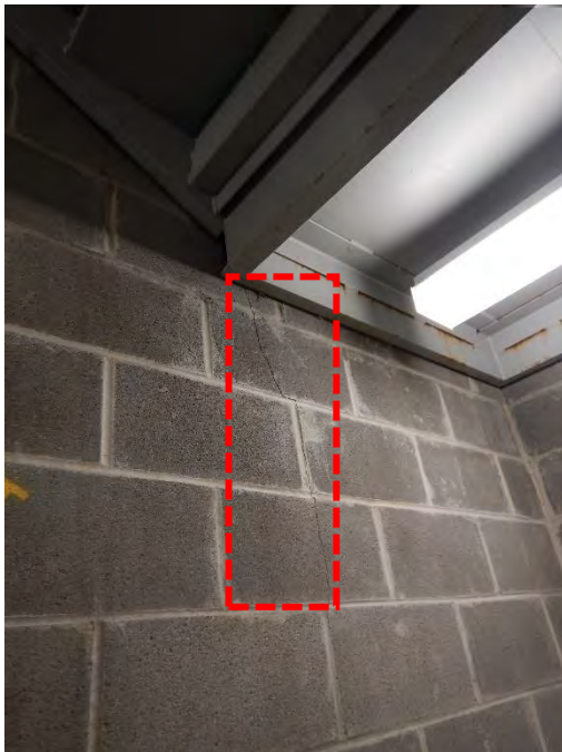
Figure 28. Cracking originating from platform connection noted in red.
