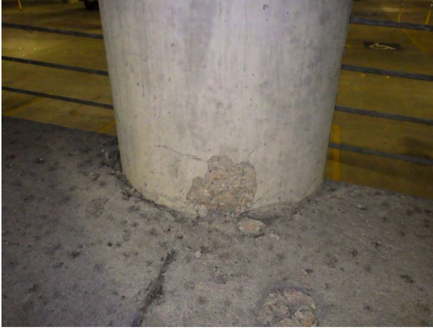
Figure 10. Observed column spalling above ramp.
