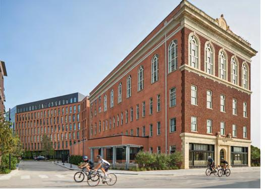
This addition has compatible proportions with the historic building and reflects character-defining elements like simple massing, brick cladding, vertical window proportions, and regularly spaced, uniformly sized window openings.
