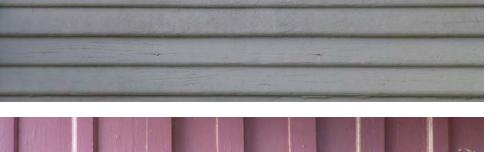
Wood is the most common type of siding in Austin, as it was easily milled into different shapes, with profiles that changed along with architectural styles.
