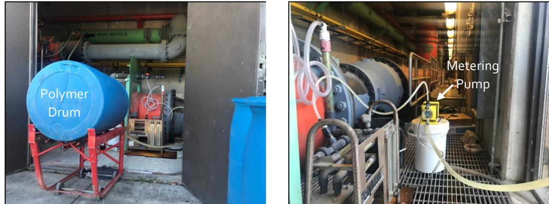
Figure 31 Demonstration-Scale Polymer Injection System
