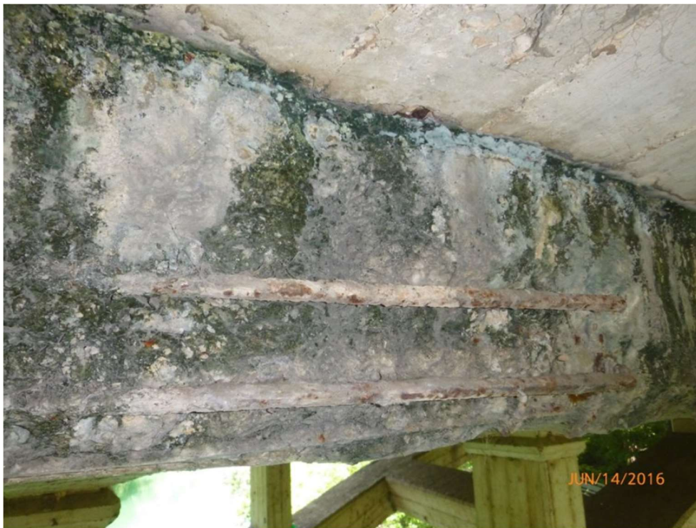
Figure 1. Deterioration of Longitudinal Beam
