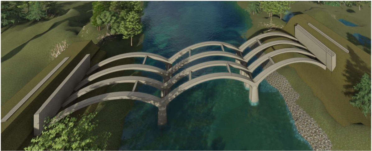
Figure 4. Bridge Rehabilitation – Remove Deck and Spandrel Columns; Remediate Remaining Structures
