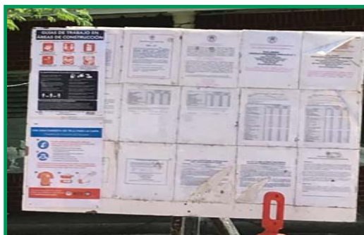
REQUIRED SIGNAGE CORRECTLY POSTED ON SITE
