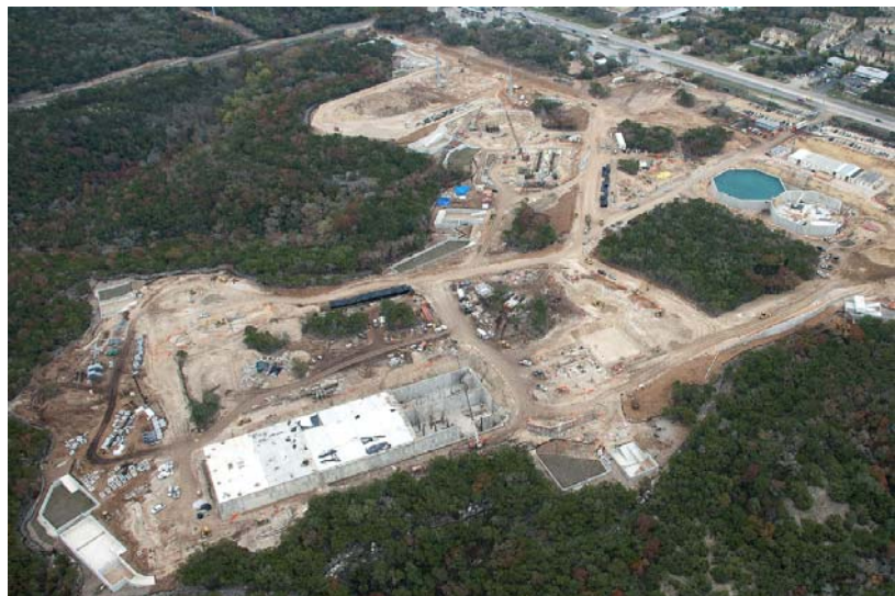
Water Treatment Plant 4 Construction Site
