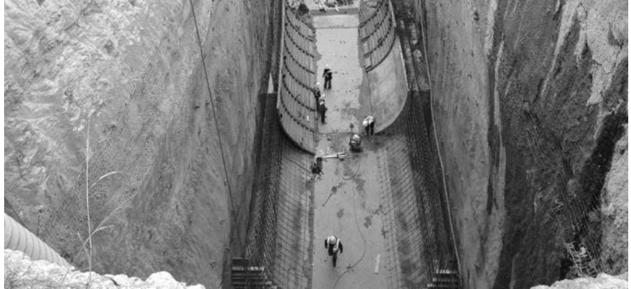
Waller Creek Tunnel Excavation
