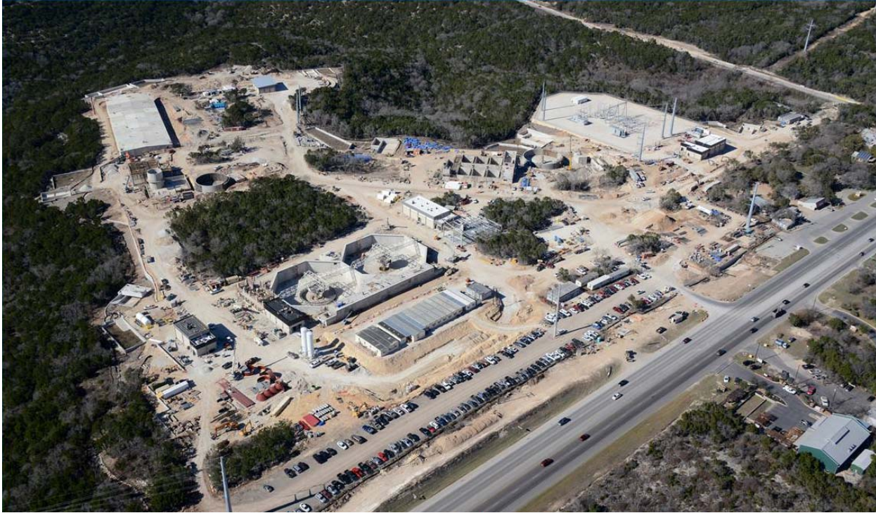
Water Treatment Plant 4 Site at Bullick Hollow
