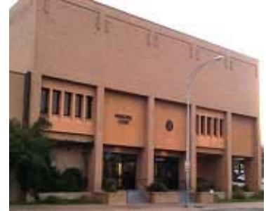
Existing Municipal Court Facility
