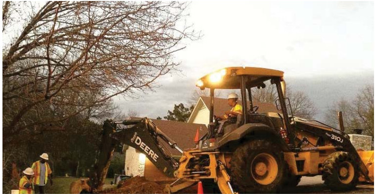
Leak Response and Repair
