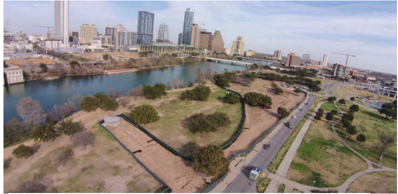
Construction at Auditorium Shores
