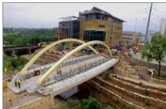
New Central Library Construction 2016
