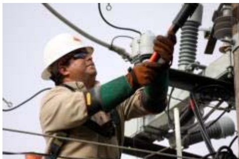
Installation of Distribution Remote Switches
