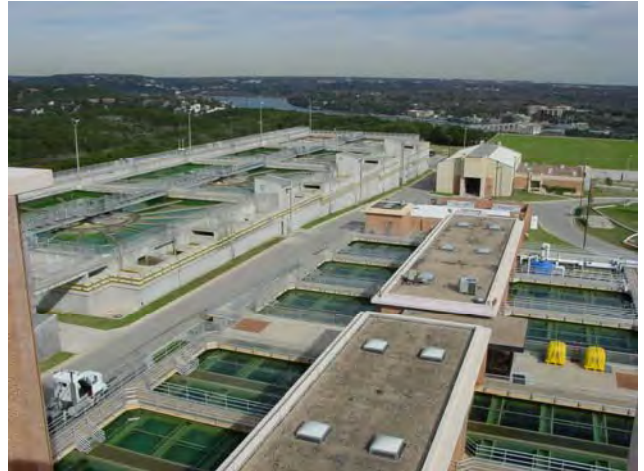
Ullrich Water Treatment Plant
