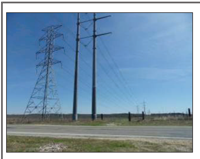
Power line easement along south boundary of Parcel 10 from Taylor Lane
