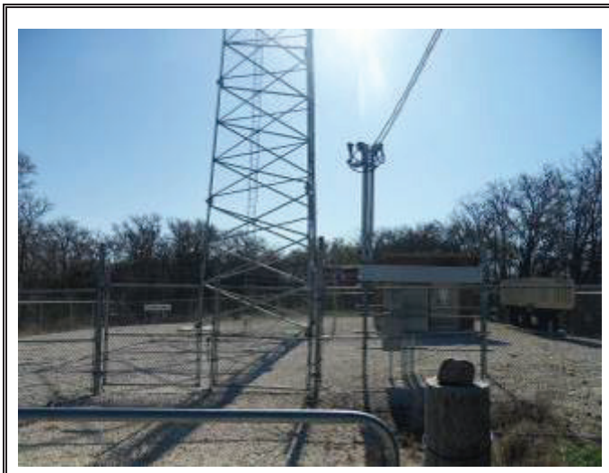
Cell tower located on Tract 2 just north of proposed Decker Lake Road
