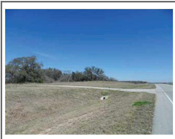
On SH-130 frontage looking north from the south end of Tract 2
