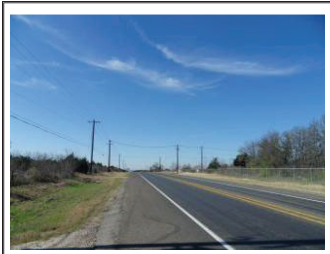
FM-973 looking south from approximately 100 yards north of intersection of FM-973 and Decker Lake Road
