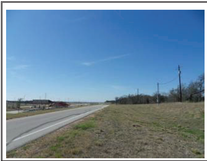
On SH-130 frontage looking south at approximate connection of Tract 1 and Tract 2 where Decker Lake Road will be built, SH-130 toll plaza can be seen to the left.
