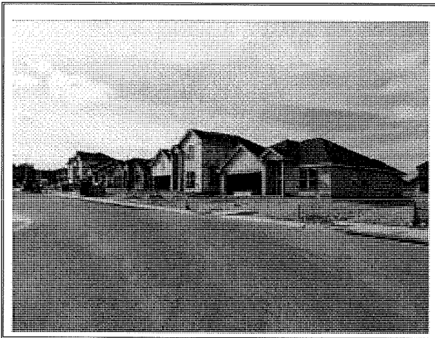
Southeast view of homes under construction (Tract 11)
