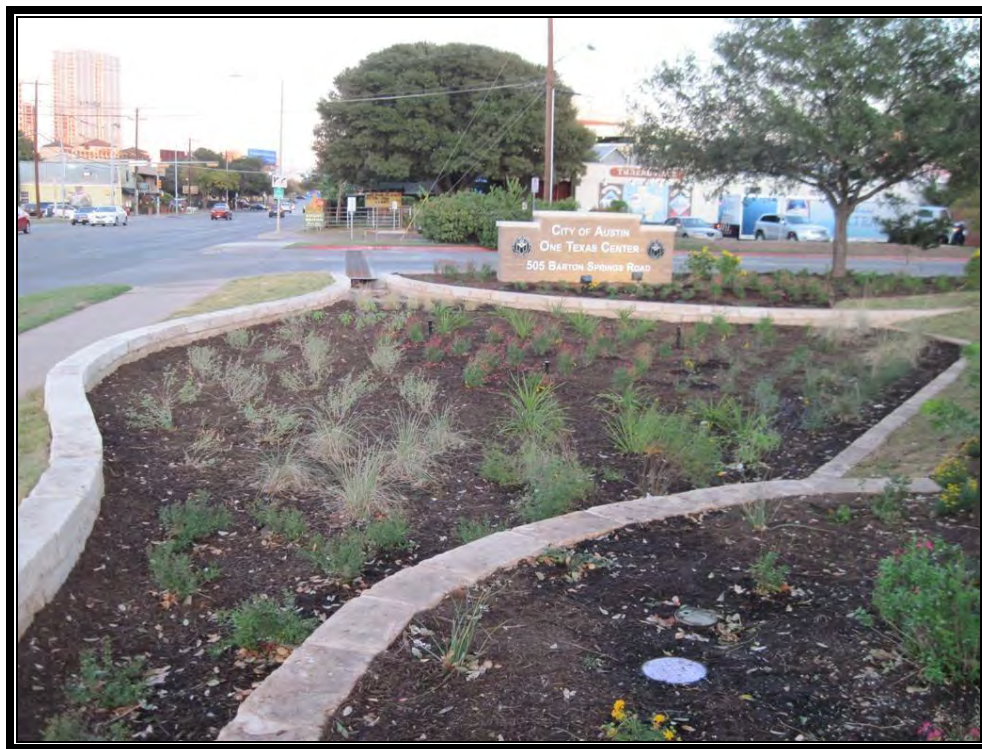
Rain garden that treats stormwater runoff from parking lot at One Texas Center
