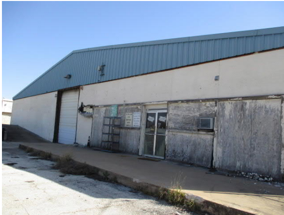
Photo 1 General view of the on-site 920 Justin Lane building
