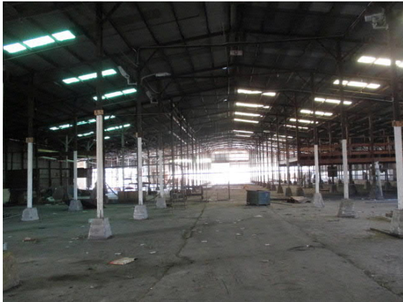
Photo 7 Additional interior view of the on-site 920 Justin Lane building
