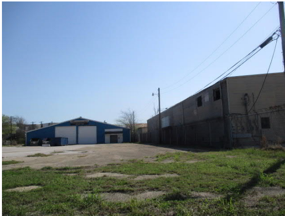
Photo 27 Properties to the northwest of the site looking east from Ryan Drive
