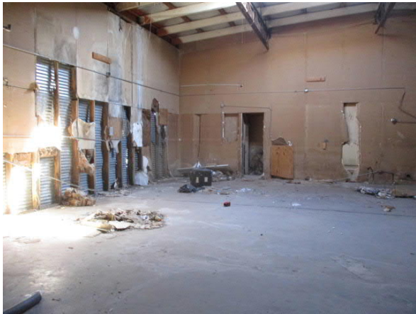
Photo 15 General interior view of the on-site 6911/6917 Ryan Drive building
