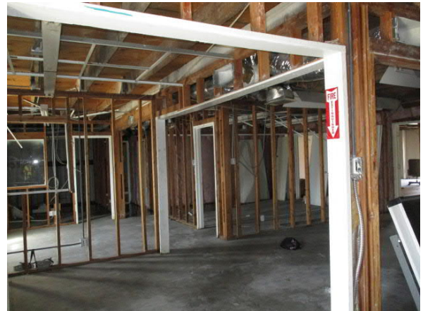
Photo 10 General interior view of the former on-site relay building
