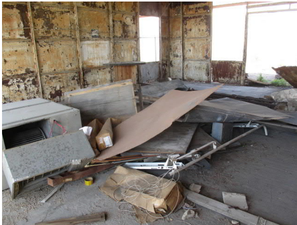
Photo 21 General interior view of the former automotive shop
