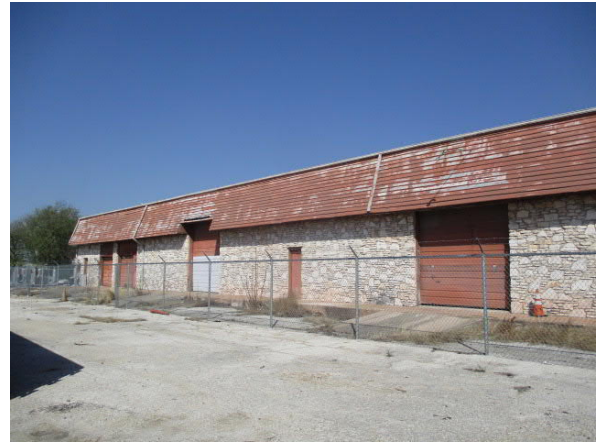
Photo 14 General view of the on-site 6911/6917 Ryan Drive building
