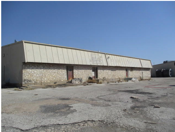
Photo 9 General view of the former on-site relay building
