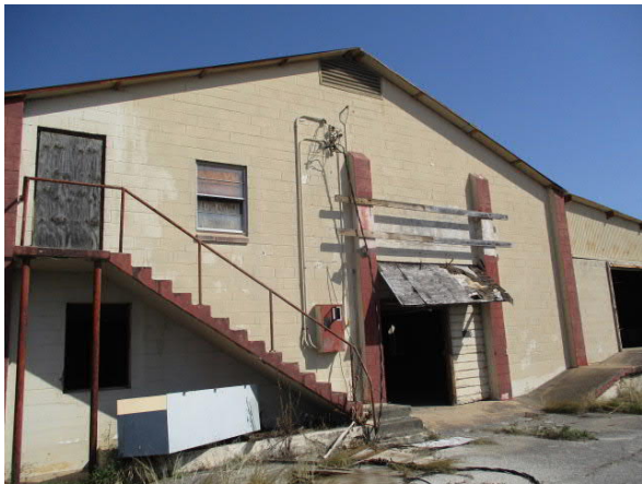
Photo 17 General view of the on-site building adjoining the 6915 Ryan Drive building
