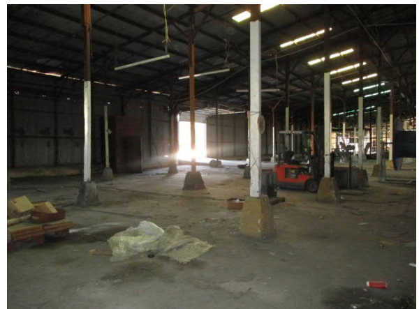
Photo 6 Additional interior view of the on-site 920 Justin Lane building
