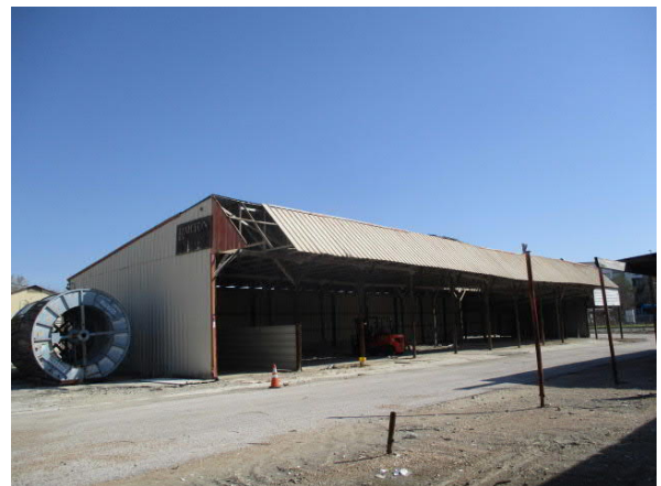
Photo 12 General view of the on-site 906/908 Justin Lane building
