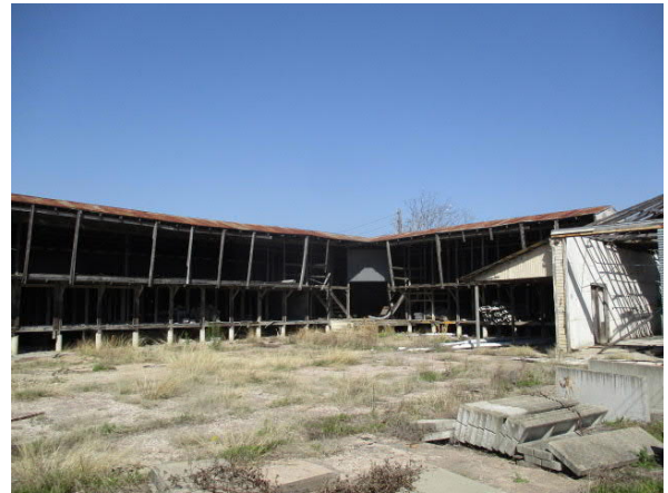
Photo 16 General view of the on-site 6915 Ryan Drive building
