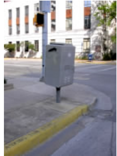
a utility box blocking a busy sidewalk creates a conflict with pedestrians
