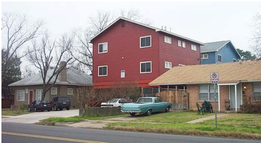
This collection of large duplexes is the type of redevelopment that neighborhood stakeholders want to discourage.
