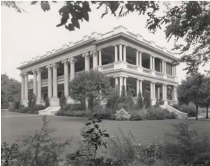
The Wooten House. Photo courtesy of the Austin History Center, PICA C01524.
