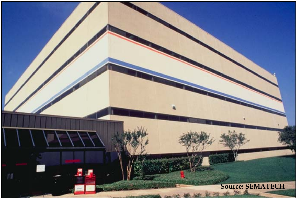
SEMATECH Administrative Building
