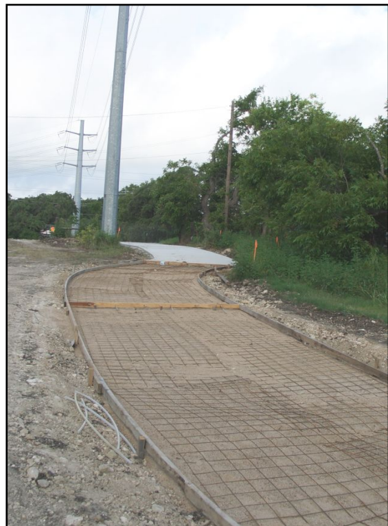
The Pleasant Valley Bikeway, seen here under construction, connects Pleasant Valley Road with Burleson Road.
