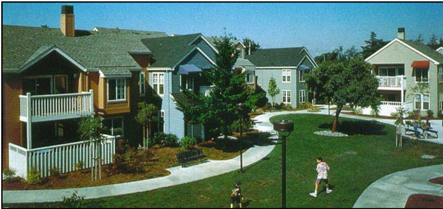
The wide, meandering path in this apartment courtyard broadens at special areas where seating is provided. ( www.designadvisor.org )
