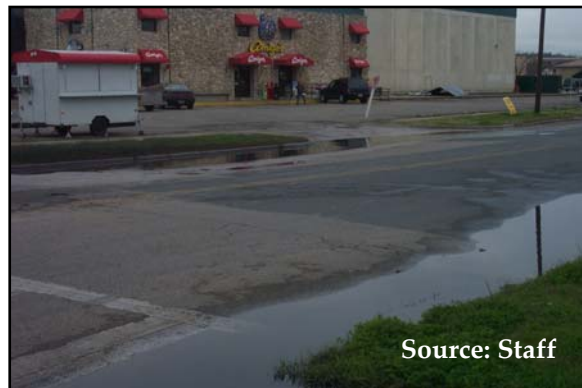
Flooding along Elmont Drive
