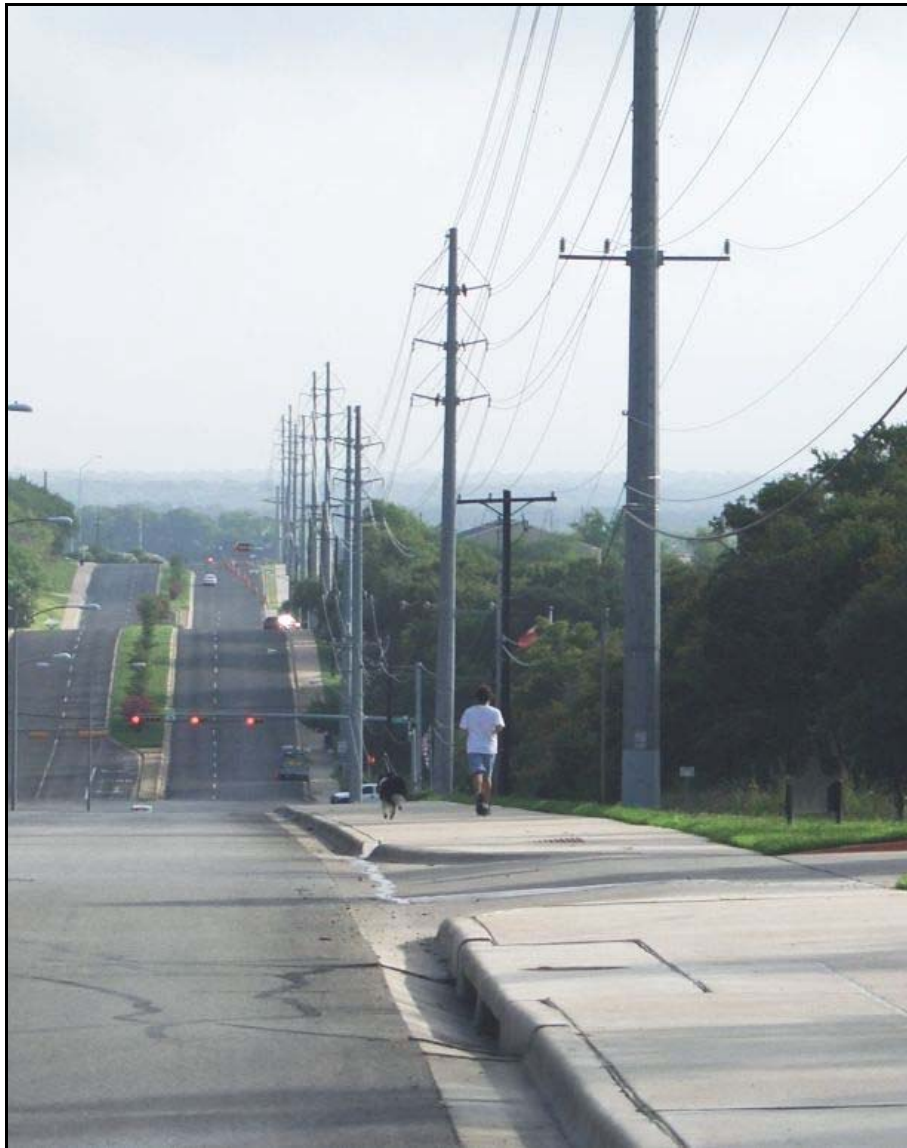
Pleasant Valley Road, looking north
