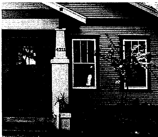
Multi-pane glazing is common to the historic styles in the neighborhood.
