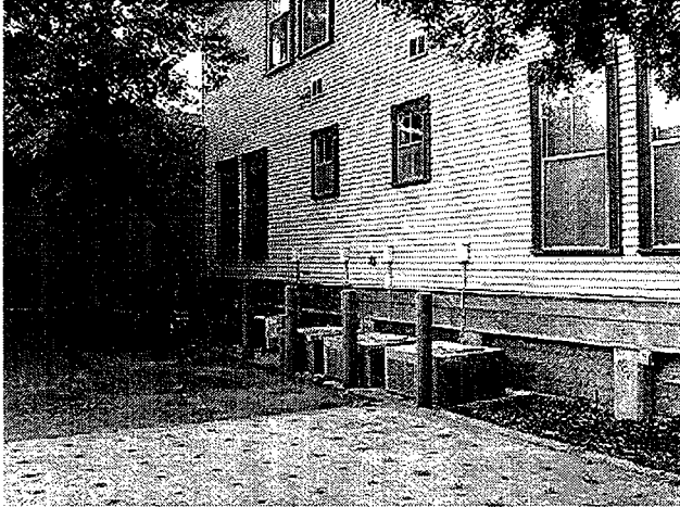
building mechanical system located behind a condominium in the neighborhood
