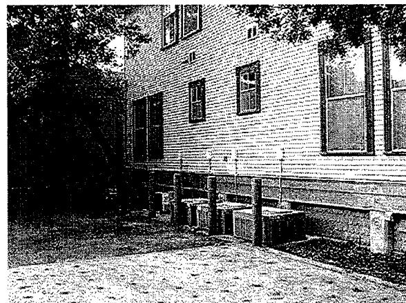
mechanical equipment at rear of building
