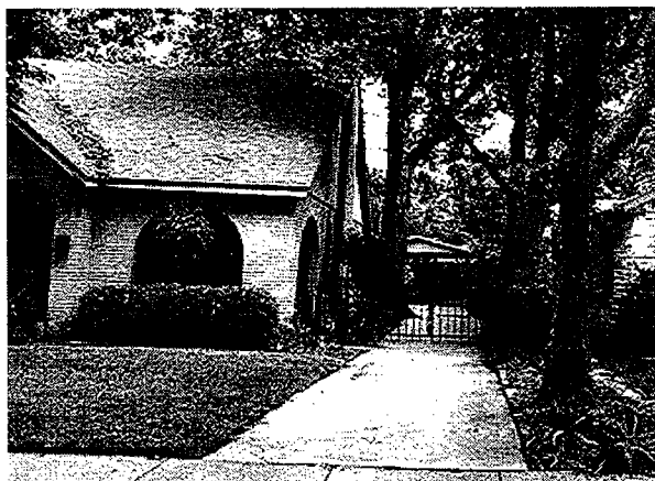
no mechanical equipment in view
