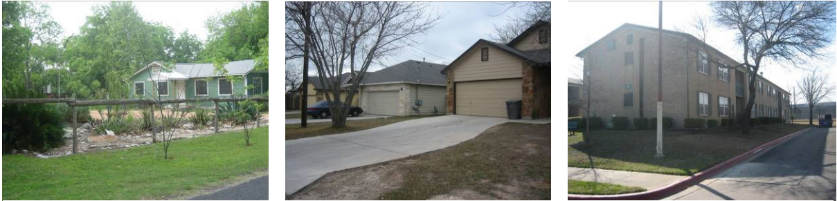
The housing stock of the NLCNPA represents its rural roots and suburban development with (from left) farm-style homes, suburban-style tract homes, and apartment complexes.
