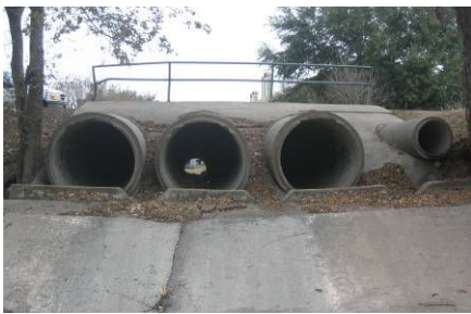
Drainage culverts underneath Masterson Pass
