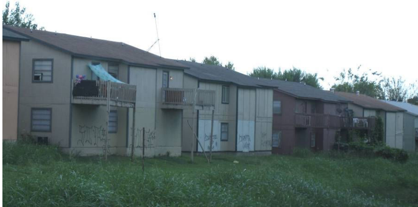
Property maintenance is lacking at the absentee landlord-owned 4-plexes on Brownie Drive.
