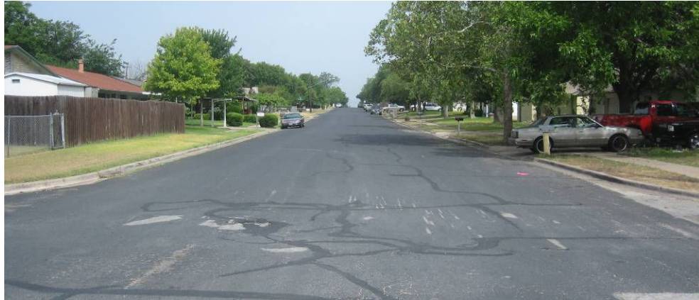
Residents on Grady Drive have reported many traffic-related issues for this residential street in the NLCNPA. Its width and lack of lane striping create hazardous traveling conditions.
