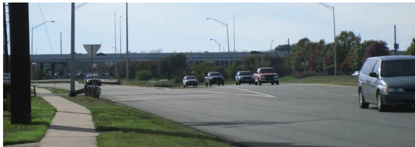
The interchange near North Lamar Boulevard and US Highway 183 is dangerous for both drivers and pedestrians.
