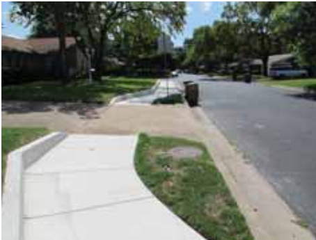
A new sidewalk segment is completed as part of the Public works Neighborhood Partnering Program.
