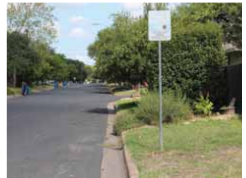
Missing sidewalk segments force people to walk on the road, putting them in danger and impairing the flow of traffic.
