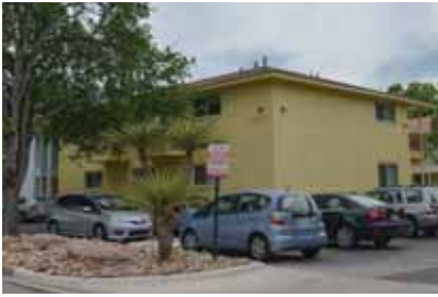
Aging apartment complexes provide affordable housing options, but could face market pressure to redevelop.
