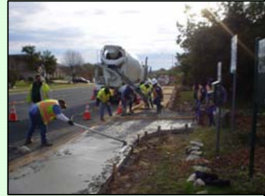
Construction of a sidewalk
