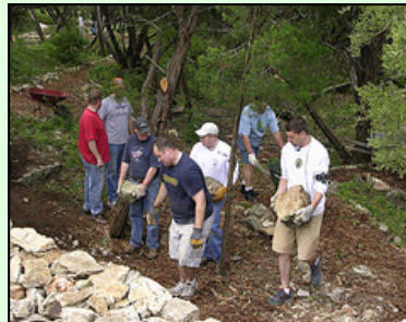
Volunteers building a stone wall
