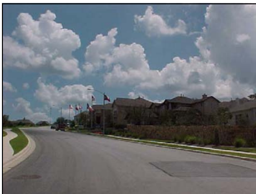
Figure 7-9: Apartments on Monterrey Oaks Blvd.
