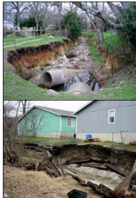
Figure 5-9: Erosion along Williamson Creek
