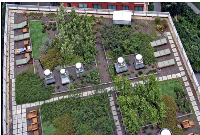
Figure 9-10: A sustainable roof
