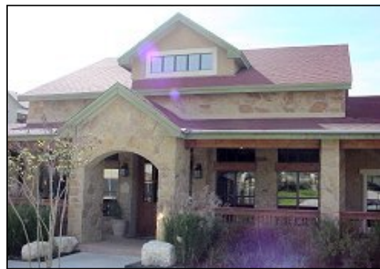
Figure 8-7: Southwest Trails, Oak Hill Photo credit: Austin Apartment Store website
