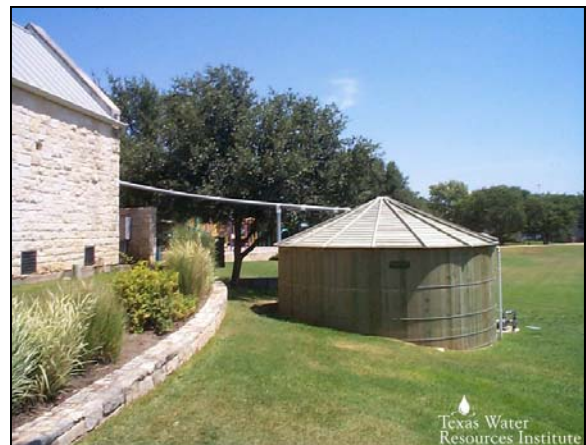
Figure 9-11: Rainwater harvesting facility
